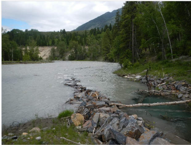
Figure 16 Aberfeldie side channel outlet and groyne under spring high flow conditions (June 7, 2013).
