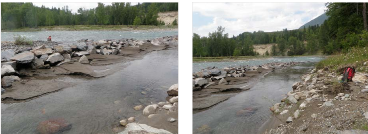
Figure 17 Sediment accumulation through rip rap at groyne after spring high flows (July 30, 2012).
