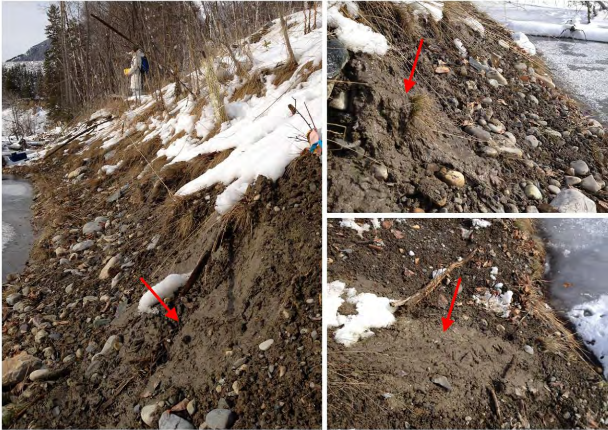
Figure 26. Erosion along slope of pool habitat unit 1-7 (right downstream boundary) of the Aberfeldie side channel (February 18, 2012). Red arrows indicate run-off of fine sediments into the channel.
