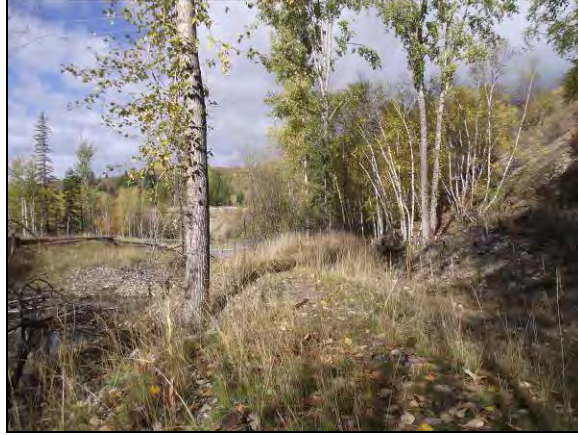
Figure 23. Berm on right downstream bank of the Aberfeldie side channel, protecting the channel from sediment input from adjacent eroding slopes (October 3, 2011).
