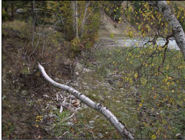
Figure 25. Bull River Bank at upstream end of the Aberfeldie side channel (October 3, 2011).
