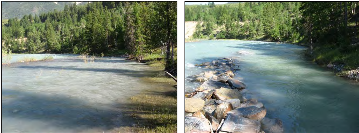
Figure 20. Side channel outlet and groyne under spring flow conditions (July 5, 2011).
