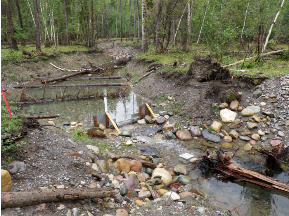
Figure 3. Image of the constructed side channel in 2009 looking upstream from the flow monitoring station. Flow in the channel at this time was 0.013 \text{ m}^3 \cdot \text{s}^{-1} .
