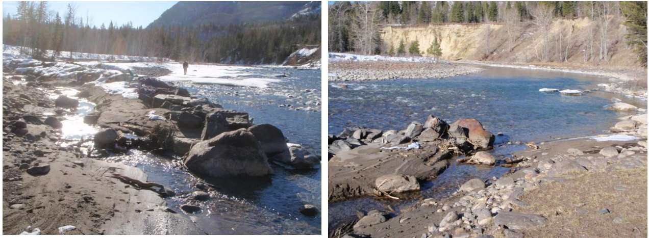
Figure 27 Upstream (left photo) and downstream (right photo) views of groyne and sediment accumulation during overwintering assessment (February 14, 2013). Side channel is open to the Bull River mainstem.
