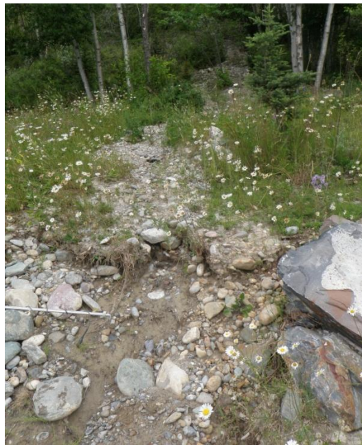
Figure 28 Erosion at right downstream berm near channel outlet (July 30, 2012).
