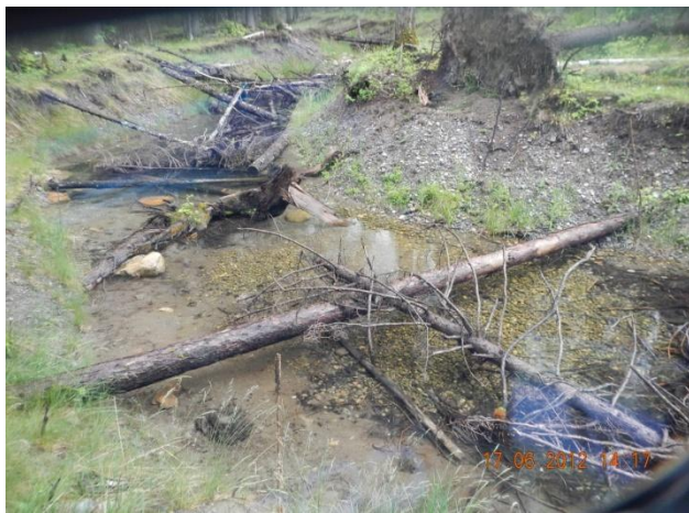
Figure 31 Erosion along slope of glide habitat unit 1-18 (upstream view) of the Aberfeldie side channel (June 17, 2012).
