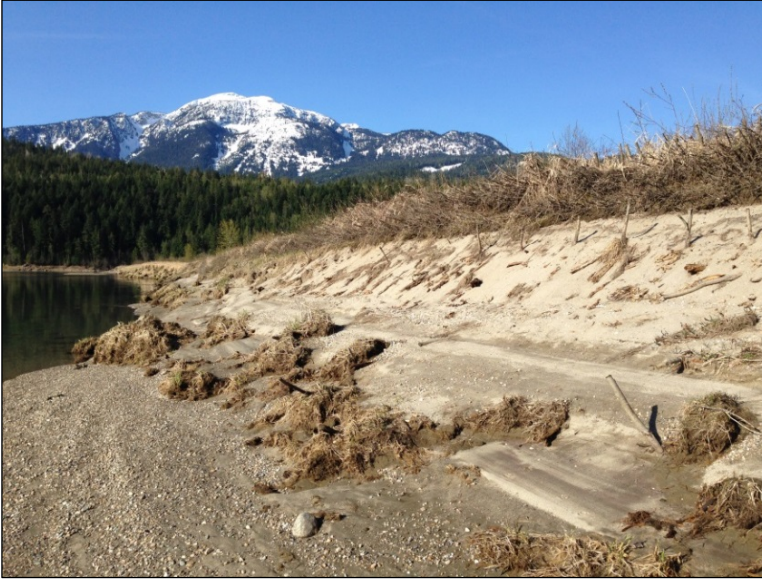
Photo 8: Site A2 Treatment Erosion of Toe and Mid-Bank, Upper Soil Wraps and Brush Layers Intact (April 21, 2015)
