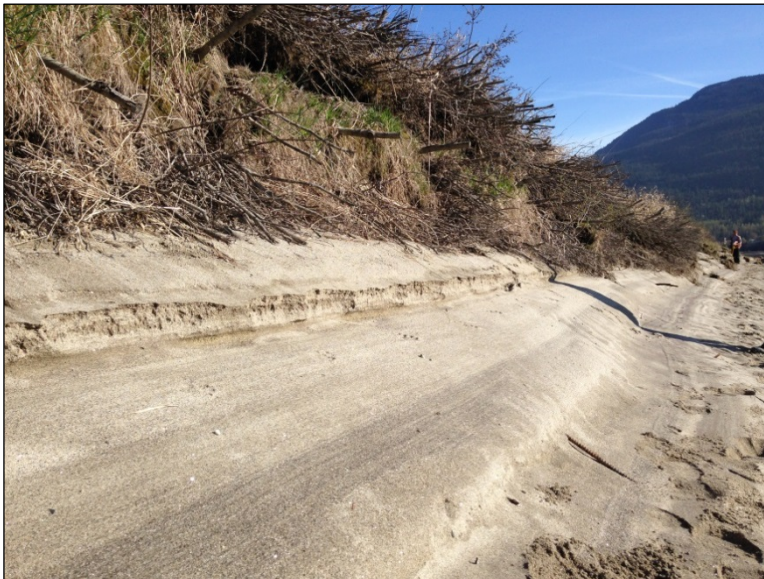
Photo 7: Site A2 Treatment Complete Erosion of Erosion Control Blanket and Willow Stakes (April 21, 2015)
