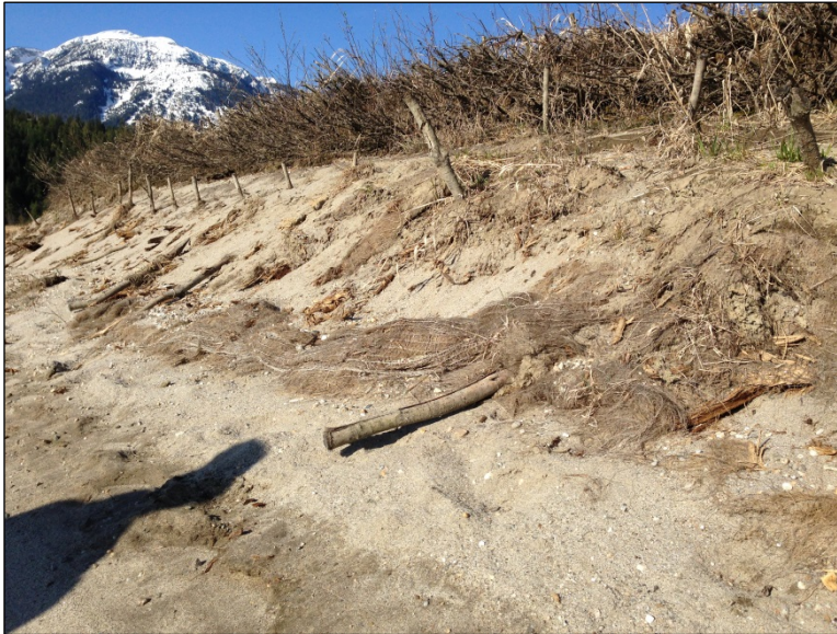
Photo 6: Site A2 Treatment Erosion of Erosion Control Blanket and Willow Stakes (Treatment Remnants Visible Mid-Photo) (April 21, 2015)
