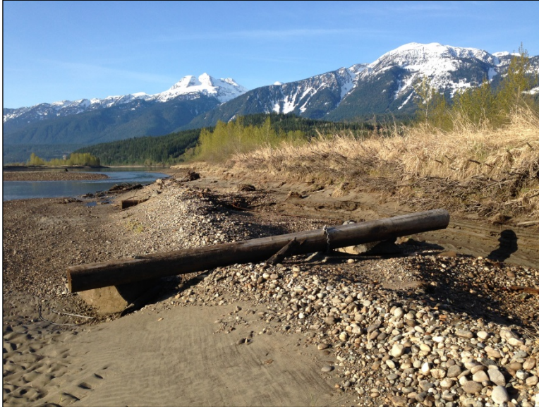
Photo 1: Site A1 Treatment Eroded Aquatic Bench, Exposed Woody Debris and Boulder Ballast (April 21, 2015)
