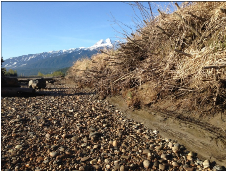
Photo 2: Site A1 Treatment Eroded Aquatic Bench, Soil Wraps and Brush Layers (April 21, 2015)
