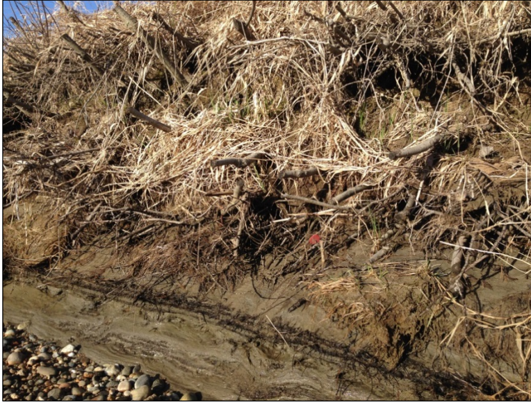
Photo 3: Site A1 Treatment Minimal New Growth of Willow Stakes and Brush Layers (April 21, 2015)
