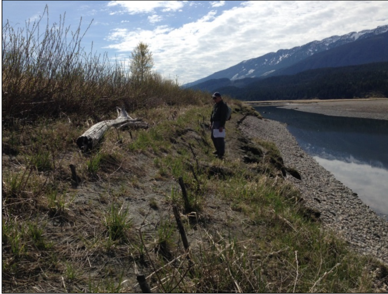
Photo 15: Erosion Control Blanket and Willow Stakes in Place Mid-Bank Toward Upstream End of Site (April 21, 2015)
