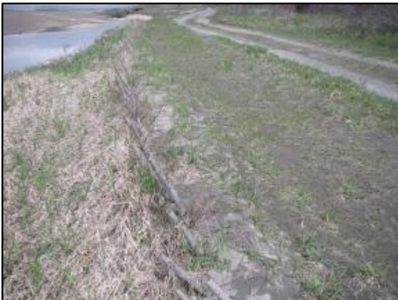
Photo 4-27 & 28: Growth in willow stakes (downstream half) and brush layer (upstream half). (April 24, 2013)
