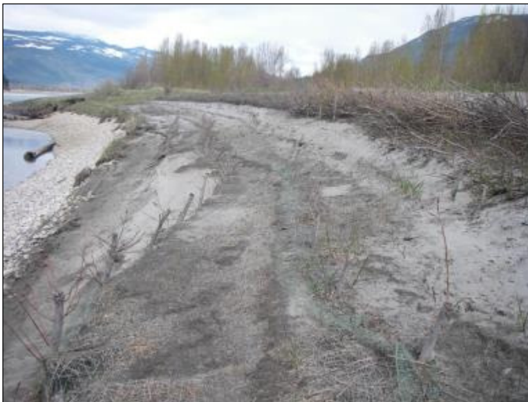
Photo 4-21: Upstream half of site, erosion of silty sand at mid bank, cocomatt and willow stakes in place. (April 24, 2013)
