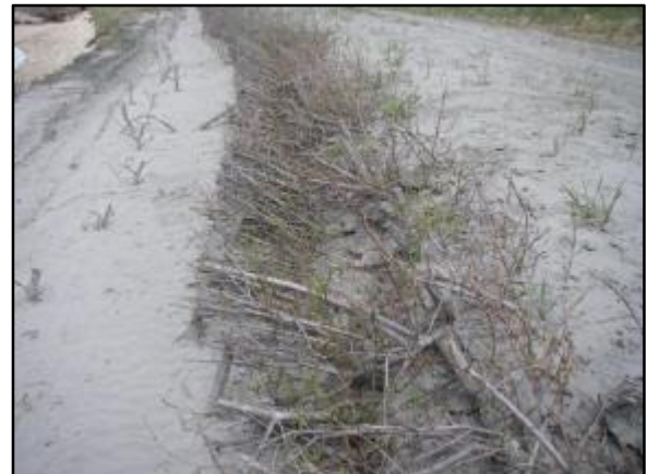
Photo 4-27 & 28: Growth in willow stakes (downstream half) and brush layer (upstream half). (April 24, 2013)
