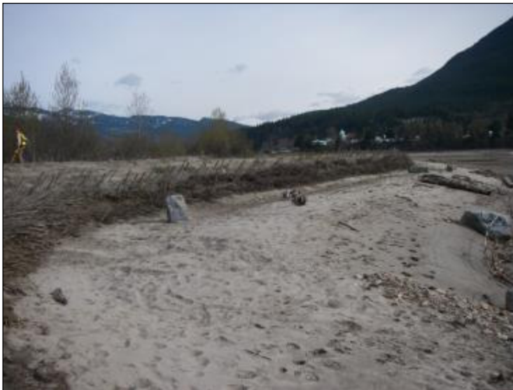
Photo 4-3: Aquatic bench at downstream end with planted grasses and sedges washed away. (April 23, 2013)
