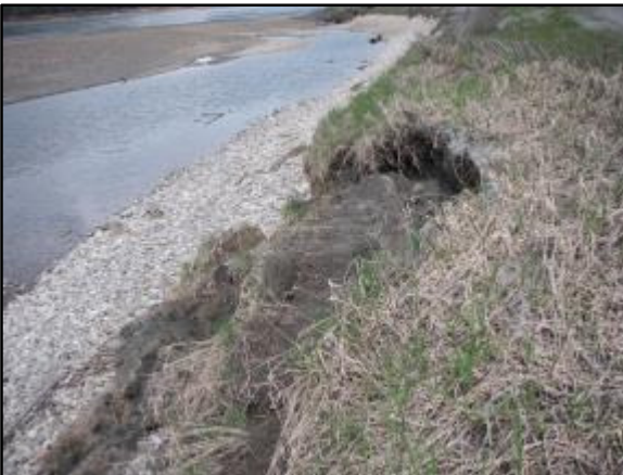
Photo 4-23 & 24: Erosion and toppling of untreated bank below brush layer (Sta. 0+700 to 710 & 0+785 to 0+805). (April 24, 2013)
