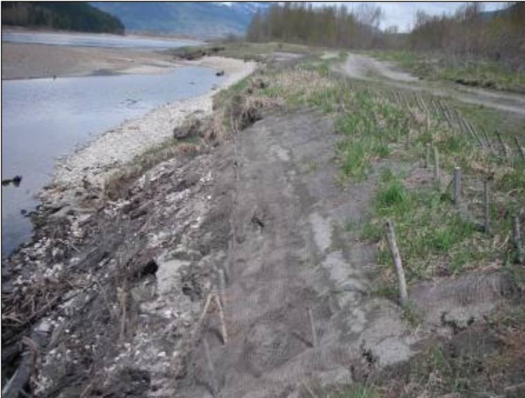
Photo 4-22: Downstream half of site, erosion at the toe of the re-graded sections in the downstream half of the site with coco-matting and willow stakes in place. Photo also shows natural deposition of woody material near the waterline. (April 24, 2013)
