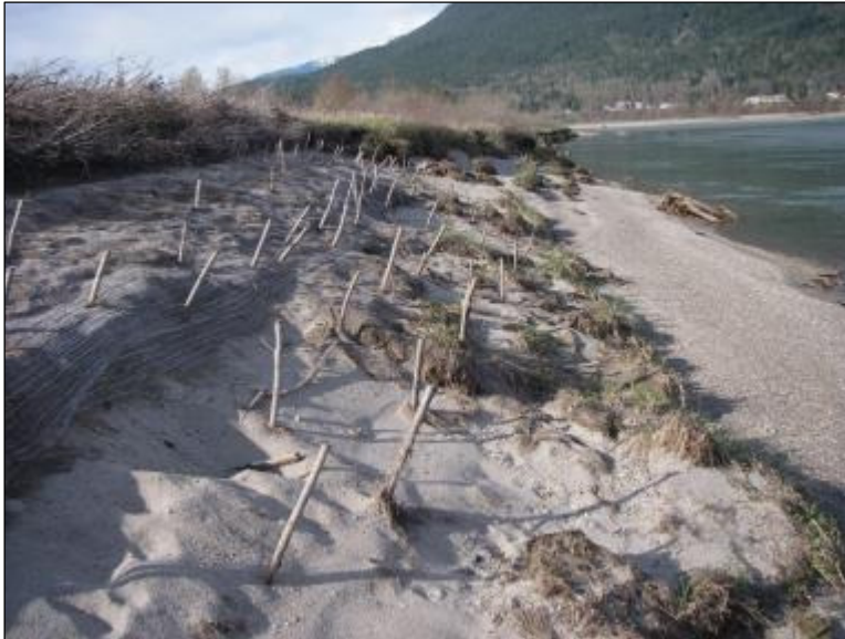
Photo 4-8: Upstream Half: mid bank with willow staking and cocomat in place. (April 23, 2013)
