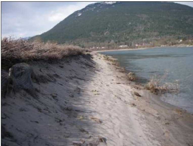
Photo 4-9: Downstream Half: mid bank with willow staking and cocomat washed away. (April 23, 2013)
