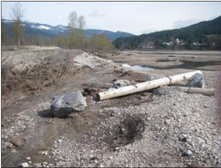
Photo 4-1: Eroded aquatic bench, exposed woody debris and boulder cluster at station 0+340. (April 23, 2013)
