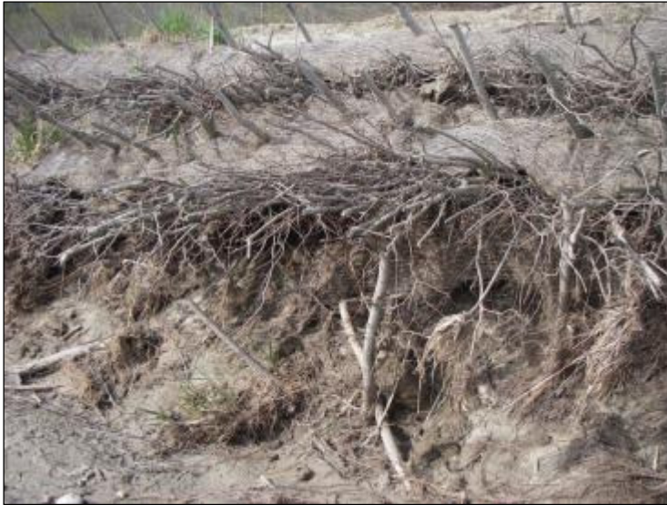
Photo 4-2: Undermined soil wraps and brush layers at station 0+340. (April 23, 2013)
