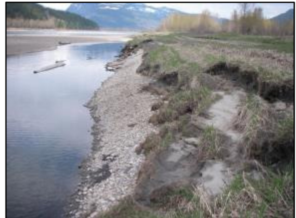
Photo 4-23 & 24: Erosion and toppling of untreated bank below brush layer (Sta. 0+700 to 710 & 0+785 to 0+805). (April 24, 2013)
