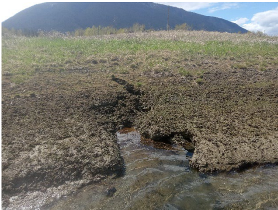
Photo 33: Erosion Feature at South End of D1, Potentially Caused by Groundwater
