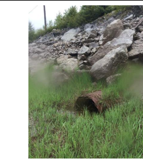
Photo 4: View of culvert outlet under Highway 6 (May 8, 2018).
