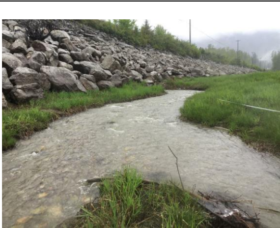
Photo 1: Upstream view at T5 (near culvert outlet) (May 8, 2018).
