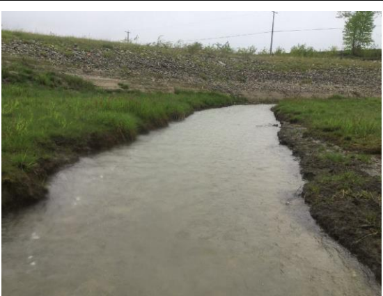
Photo 6: Downstream view at T4 (May 8, 2018).
