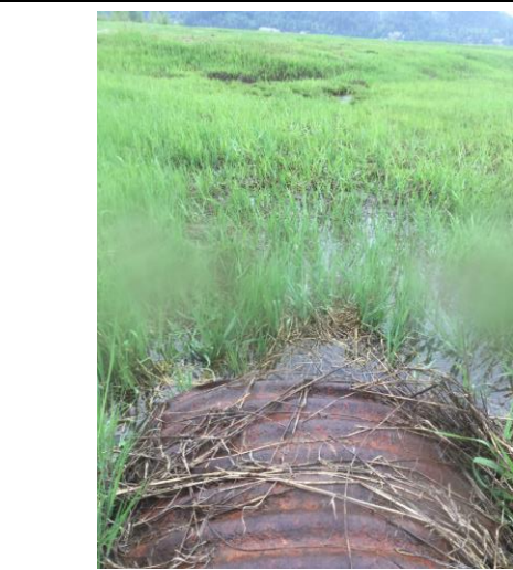
Photo 3: Downslope view of culvert outlet within non-defined channel section (May 8, 2018).
