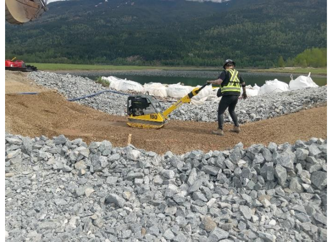
Photo 6: Preparation of the subgrade for the ACBM's at the Site 15a outlet in progress. Looking east. May 8, 2023.
