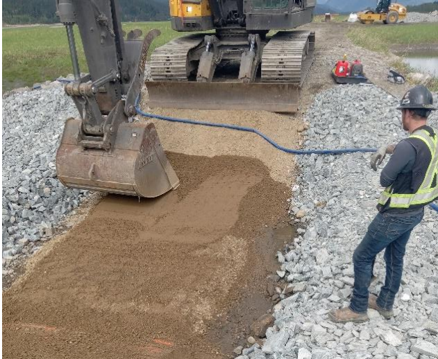
Photo 5: Preparation of the subgrade for the ACBM's at the Site 15a outlet in progress. Looking north. May 8, 2023.
