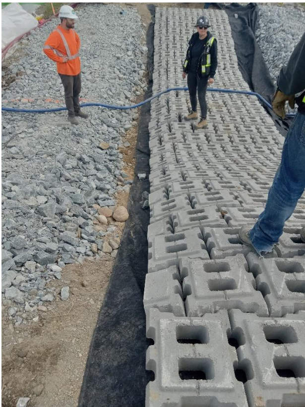
Upstream row of blocks on slope (to be embedded with 200 mm minus granular fill), looking south:
