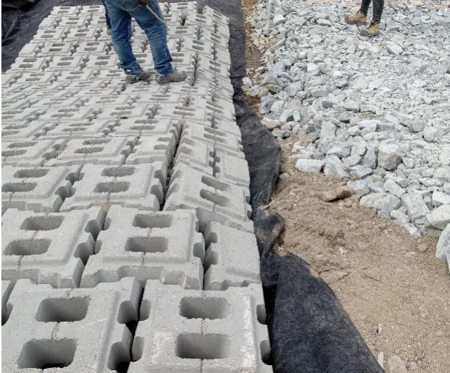
Photo 9: The first ACBM after placement. The upstream/eastern row of blocks was placed on an angle for embedment in granular material. Looking north. May 8, 2023.
