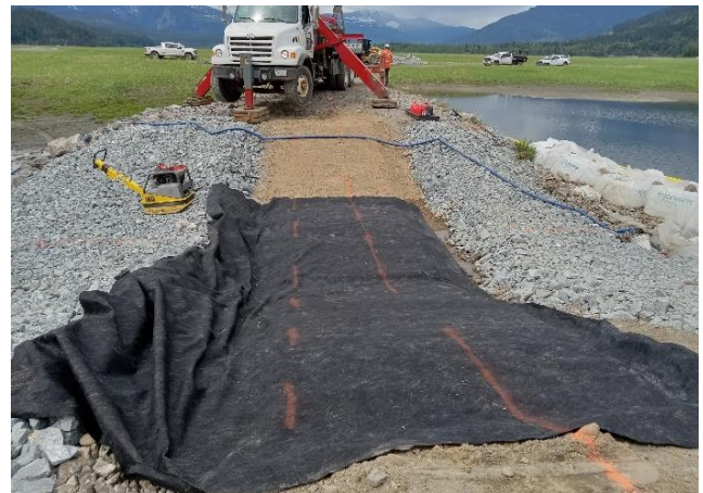
Photo 8: Placement of geotextile over the subgrade prior to placement of the first ACBM at the Site 15a outlet. Looking north. May 8, 2023.
