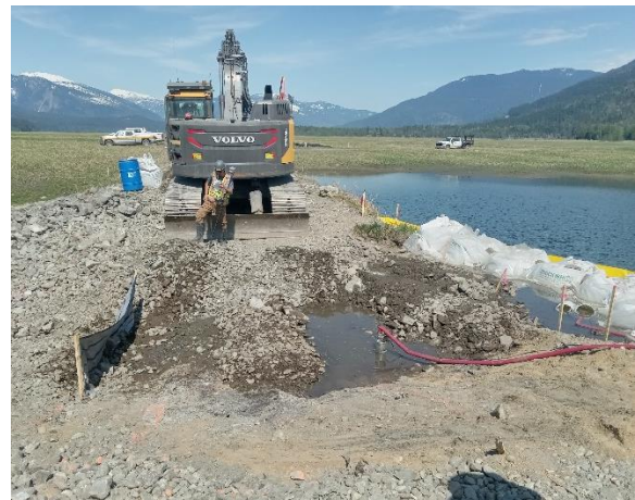
Photo 4: Excavation of the Site 15a outlet in progress. The cofferdam can be seen to the left in the photo. Looking north. May 4, 2023.
