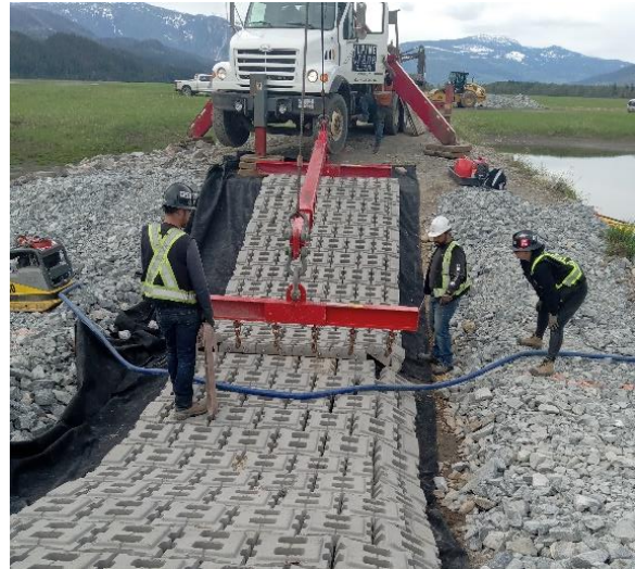
Photo 10: Placement of the second ACBM to contact the first in the middle of the Site 15a outlet. Looking north. May 8, 2023.
