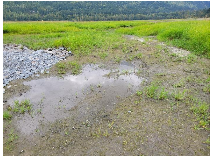
Photo 18: South end of the saddle dam where flow was observed flanking it. The area is still predominantly bare of vegetation. September 25, 2023.
