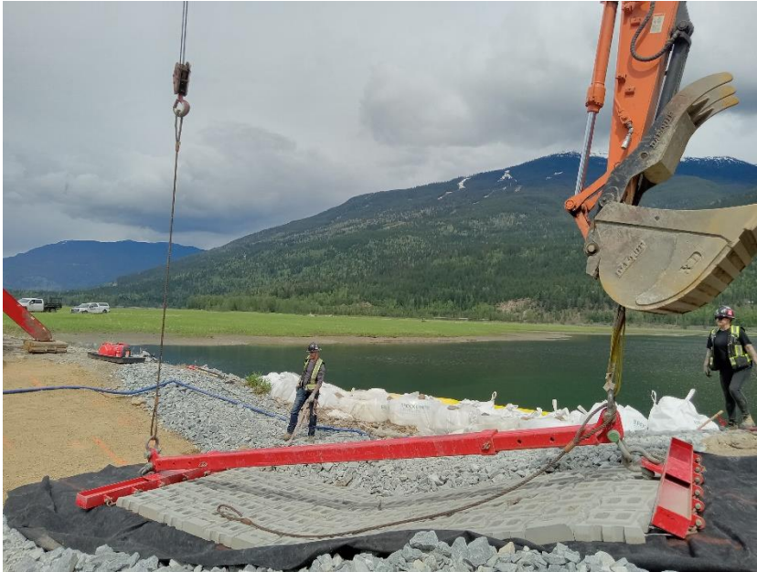
Crane and excavator placing south ACBM, looking east:
