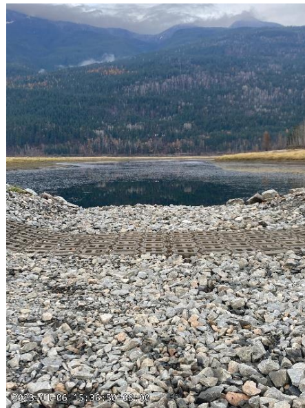
Photo 20: Wetland side of Site 15a inlet filled to provide a more uniform surface across its length. November 6, 2023.
