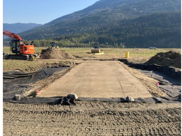
Photo 2: Placement of saddle dam fill at Area B saddle dam. Looking east. May 3, 2023. Photo provided by BC Hydro
