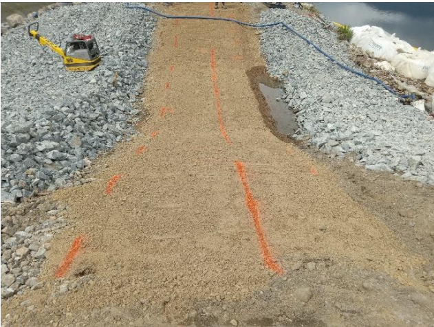
Photo 7: Finished subgrade prior to placement of the ACBM's at the Site 15a outlet. Looking north. May 8, 2023.
