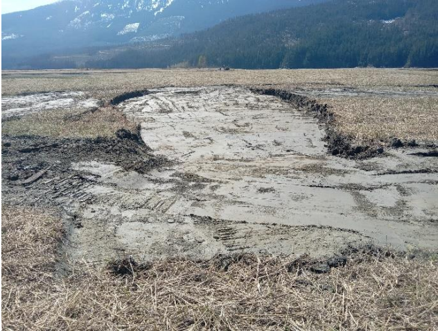
Photo 1: Excavated saddle dam footprint and prepared subgrade at Area B saddle dam. Looking west. April 30, 2023.
