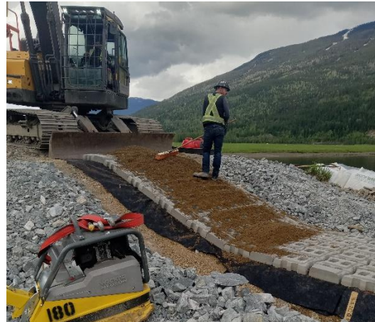
Photo 12: Filling the ACBM open cells with 25 mm minus surfacing aggregate at the Site 15a outlet. Looking northeast. May 8, 2023.
