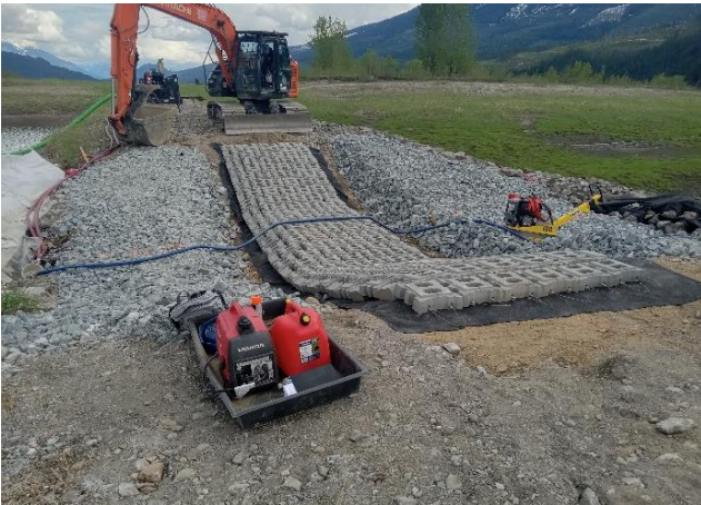
Photo 11: Both ACBM's at the Site 15a outlet in place prior to covering with surfacing aggregate. Looking south. May 8, 2023.
