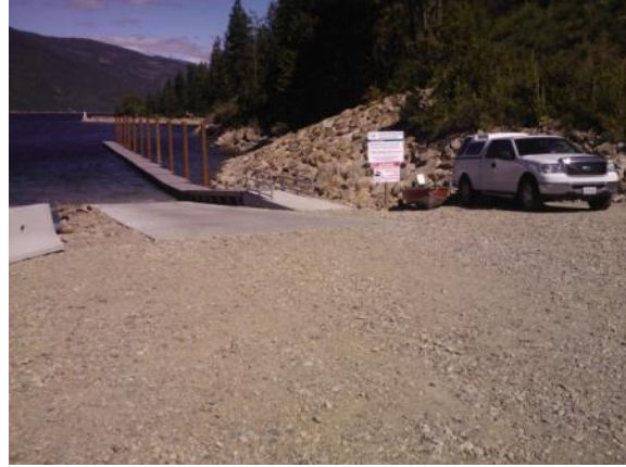
Figure 21. Anderson Point after
