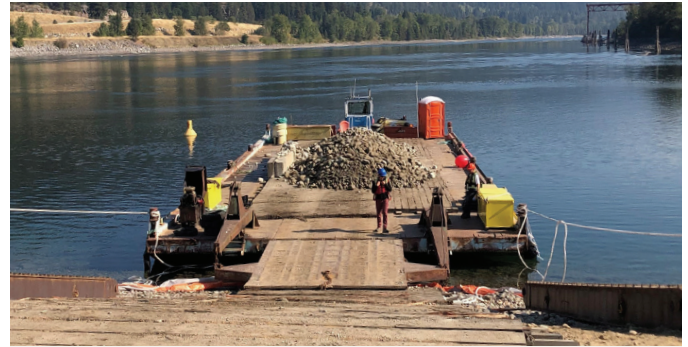
A specific mix of rocks and gravel will improve conditions for incubating eggs and larvae in the tailrace of Arrow Lakes Generating Station. Photo by Margo Sadler.
