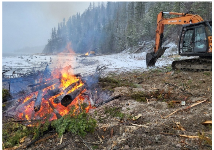
Shore-based debris removal at Van Houten Creek.
