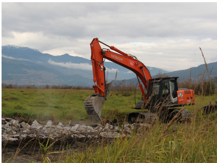
Placing rock rip rap to protect the airport slough wetland near Revelstoke.
