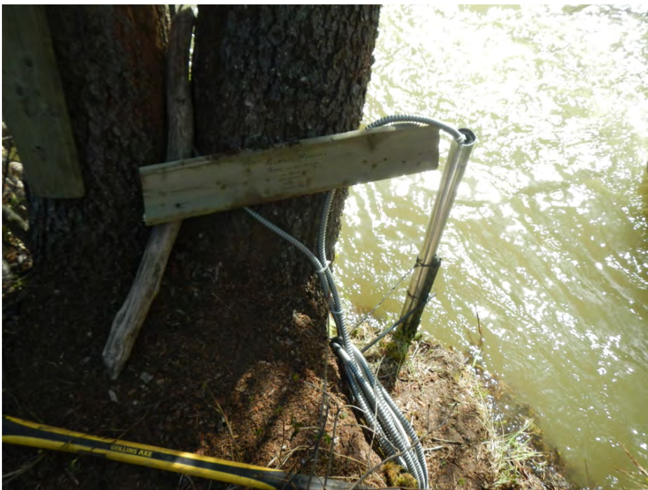
Photo 1. Housing for water level and temperature probe at Six Mile Creek gauging station.
