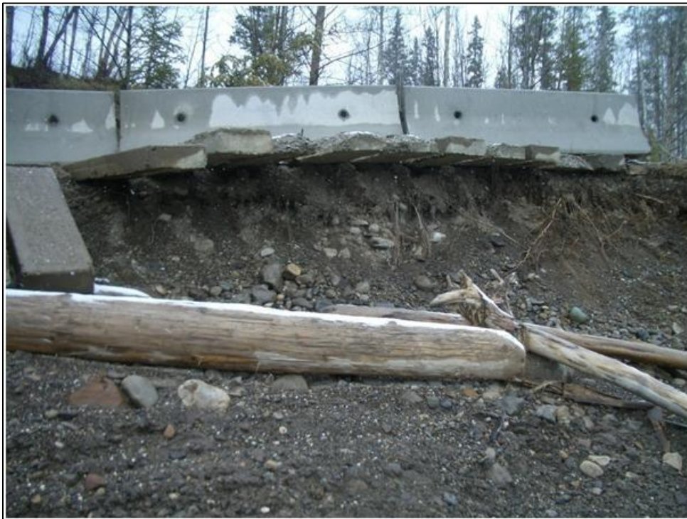
Photo 4: Taken on 5-19-2009 at Existing Dunlevy Site (Erosion and undercutting of the upper part of the existing boat launch ramp; concrete barrier has been installed for safety).
