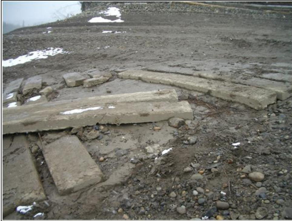
Photo 5: Taken on 5-19-2009 at Existing Dunlevy Site (Bank slumping and associated damage of the lower part of the existing boat launch ramp).
