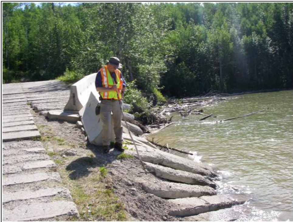
Photo 8: Taken on 7-12-2012 at Existing Dunlevy Site (Erosion damage to concrete panels at the existing boat launch ramp).
