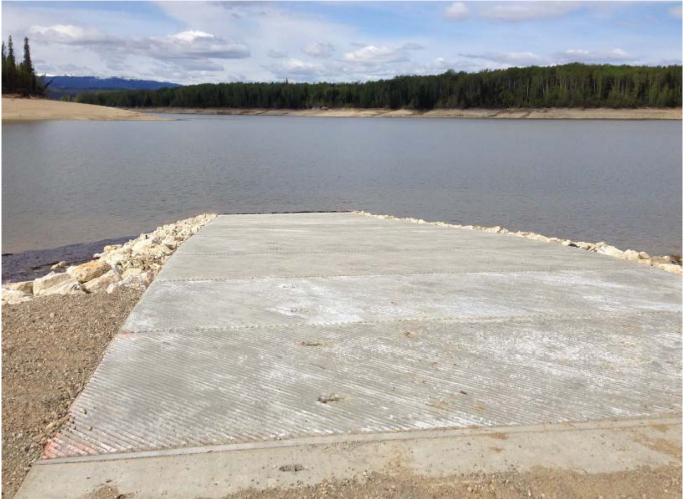
View of low water ramp and portion of turnaround area
