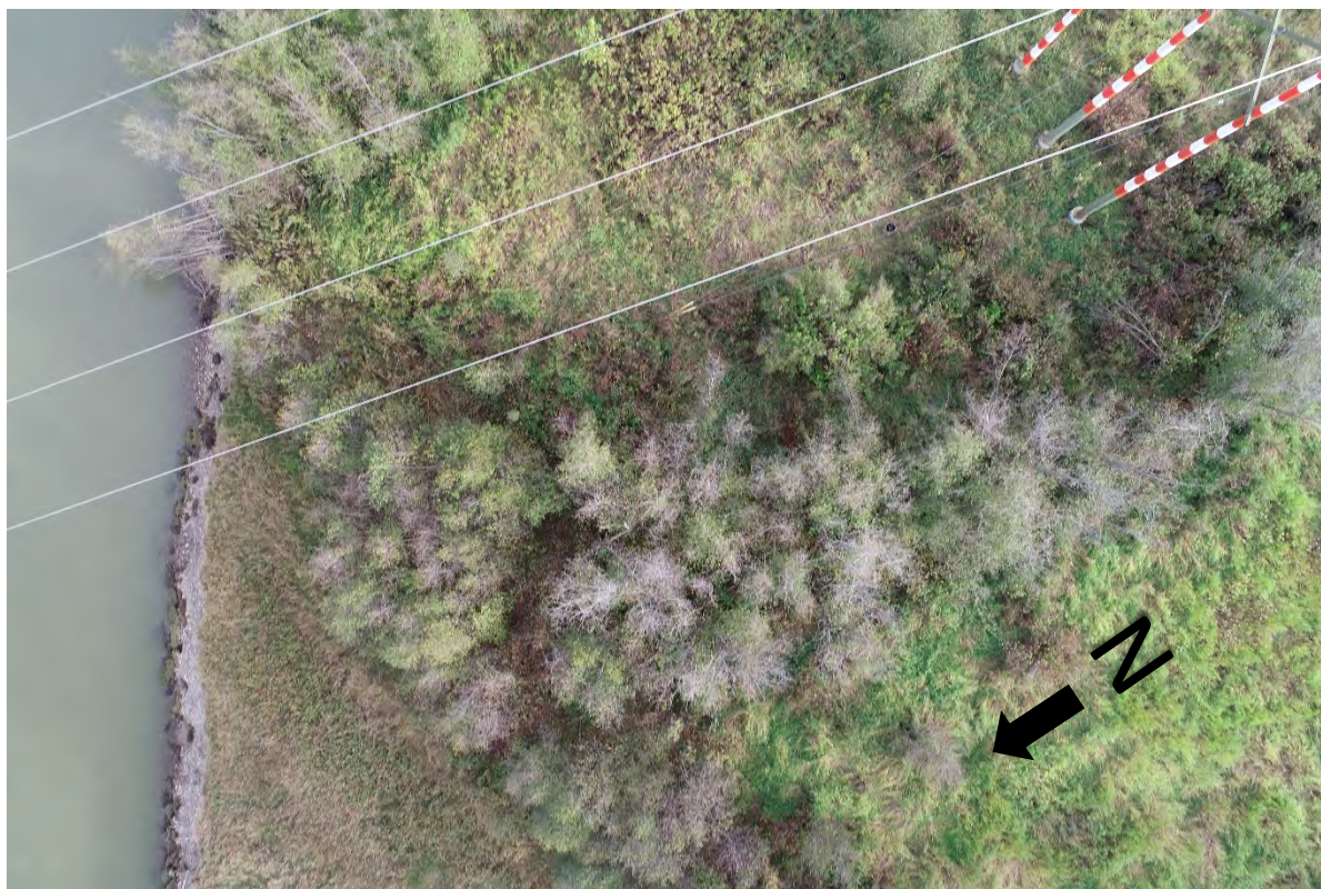
Photo 22 Drone photo of BC Hydro utility towers and eroding right (south) bank of Peace River (north side of island)
