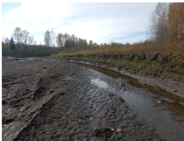
Photo 14 Section 1.5, view south west of right bank erosion
