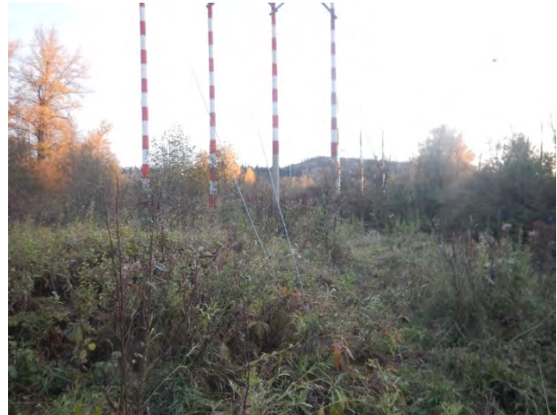
Photo 26 View of BC Hydro utility towers
