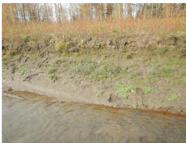
Photo 16 Section 1.5, right bank erosion
