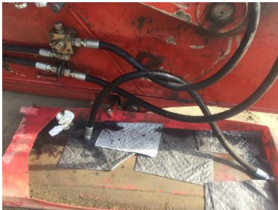
Figure 33 : Managing and replacing leaking hoses with spill kit and tray.
