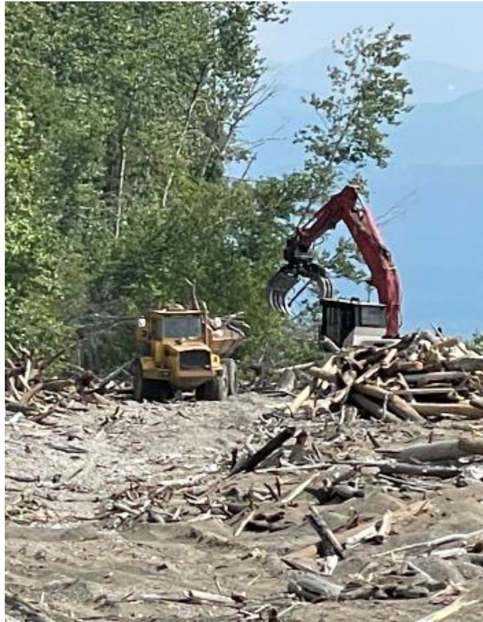
Figure 14 : Debris piling by Link Belt on Peace Point beach
