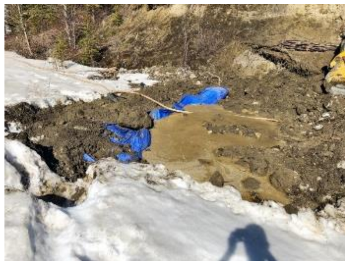
Figure 30 : Creating the berm for the Inverted Culvert
