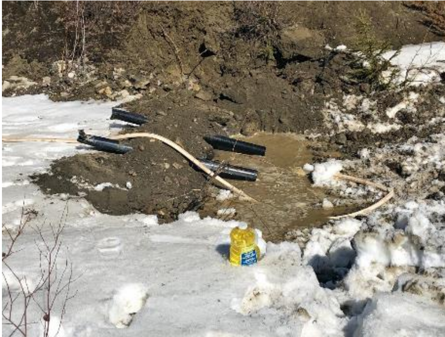
Figure 31 : Completed Inverted Culvert for the course
