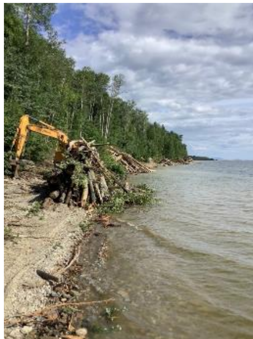
Figure 18 : Debris piling by excavator on North Bevel Beach.
