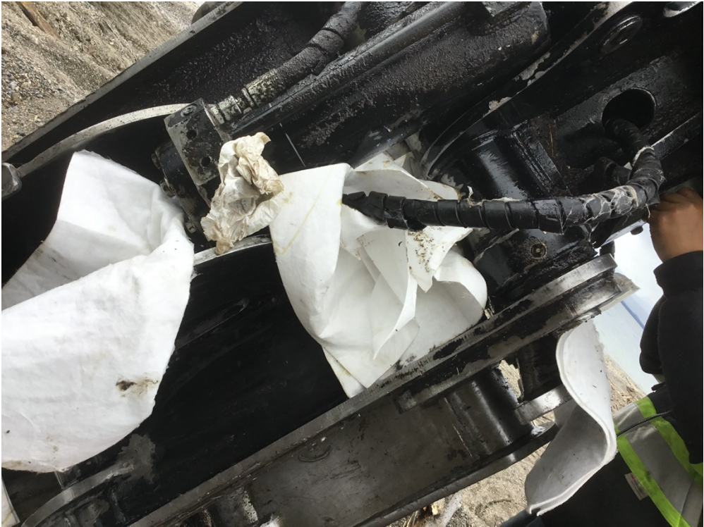
Figure 16: Managing and replacing leaking hoses with the spill kit.
