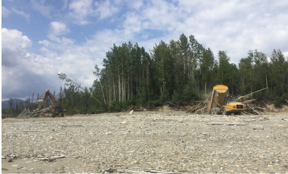
Figure 11: Debris piling by excavator and rock truck on Corless Beach.
