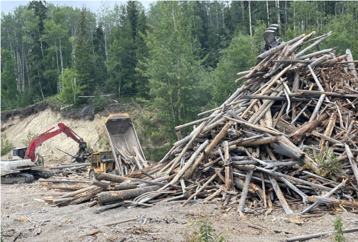
Figure 9 : After Debris piling Bevel
