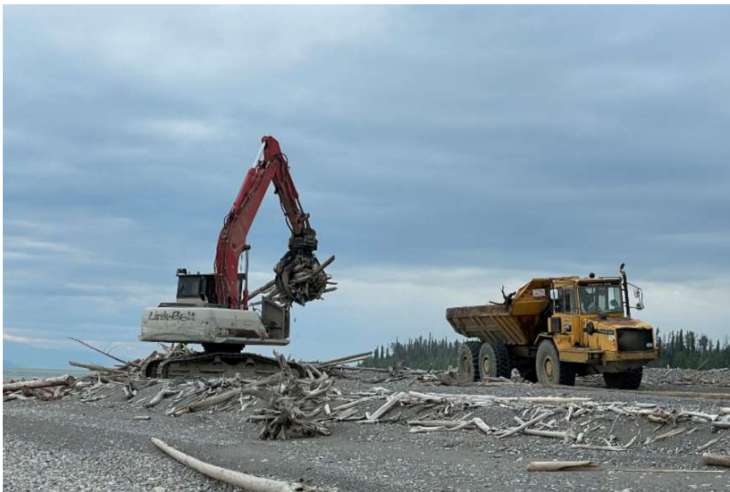
Figure 6: During Debris piling on Coreless
