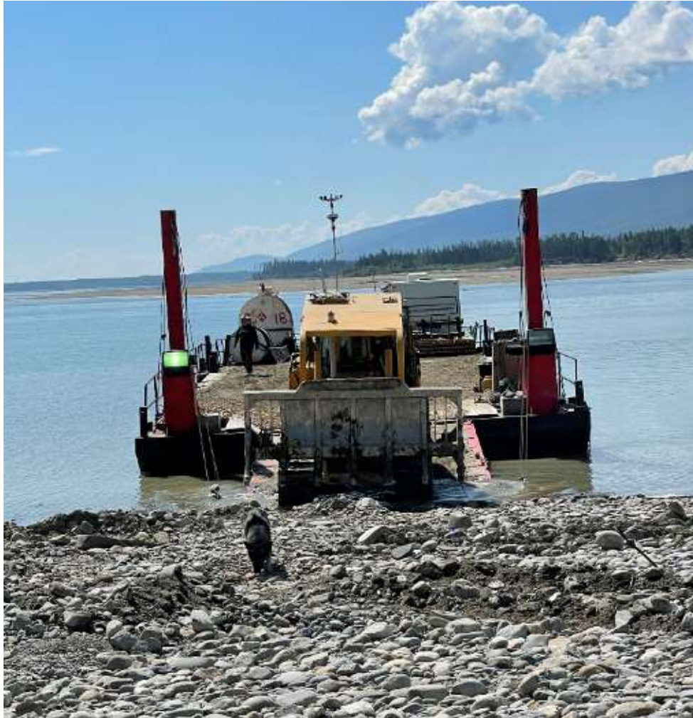
Figure 1 : Dozer being unloaded from barge
