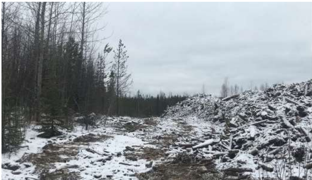
Figure 24: Assorted After Debris Cleanup Deserter's Dump-fireguard between timber and debris pile (from previous years)
