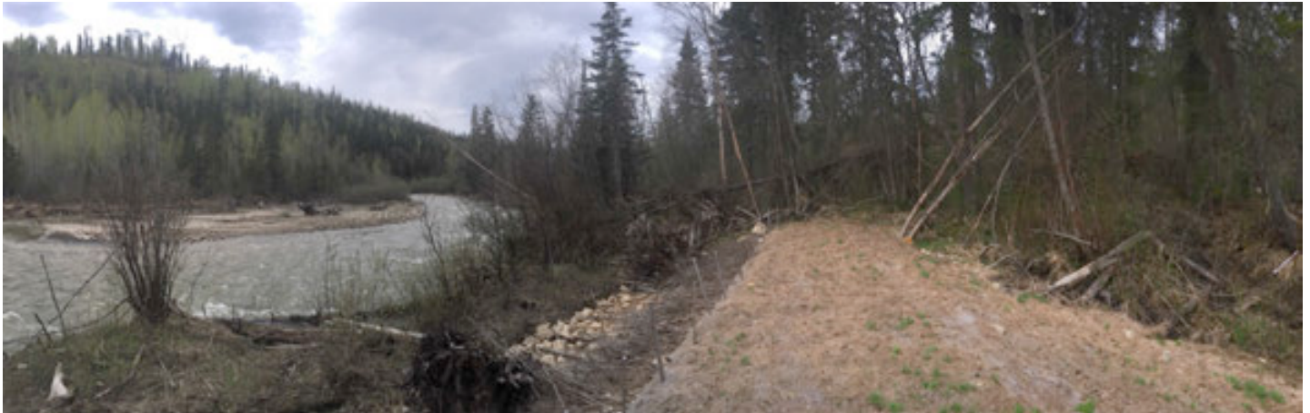
PHOTO 45 (Panoramic): Upstream end of Berm 'J' looking upstream
