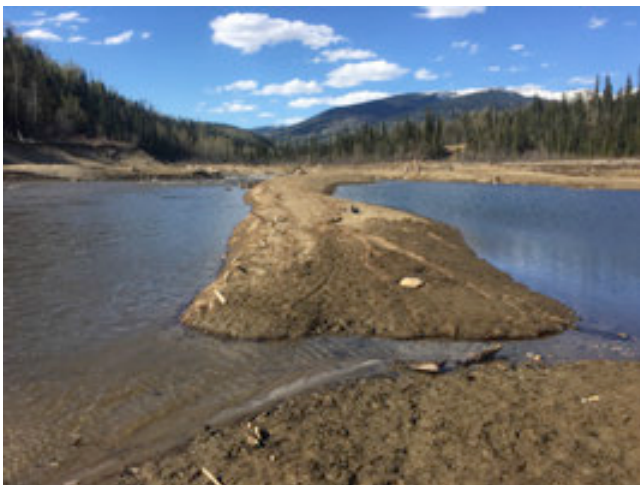
PHOTO 12: Downstream End of Berm 'F' Looking Upstream. Possible Erosion Downstream of Berm in 'Natural' Area (Note Water Flowing from Left to Right Side of Photo).
