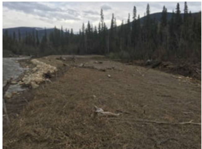
PHOTO 41: Looking upstream at upstream end of Berm 'C', note flotsam deposition from reservoir in 2015 indicating that the berm was likely mostly submerged in 2015. Note 2015 grass growth.
