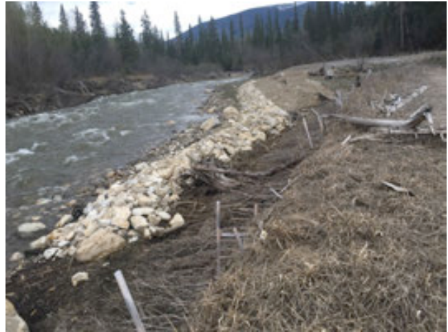
PHOTO 39: Looking upstream at willow layers (mostly dead) in the lower berm and grasses in the upper berm that had grown (not active growth yet this year given time of site visit).
