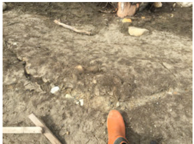
PHOTO 5: Ice Damage to ECM.
