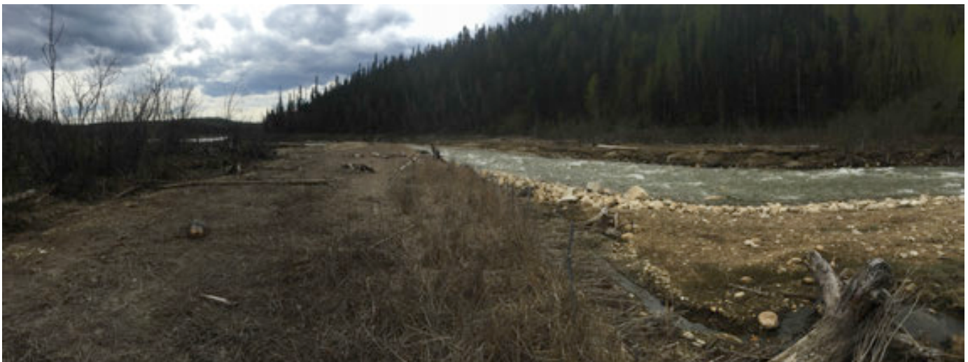
PHOTO 32 (Panoramic): Looking downstream from upstream end of Berm 'C'
