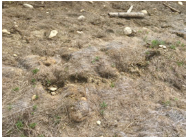
PHOTO 55: Moose related damage on back-side slope of berm
