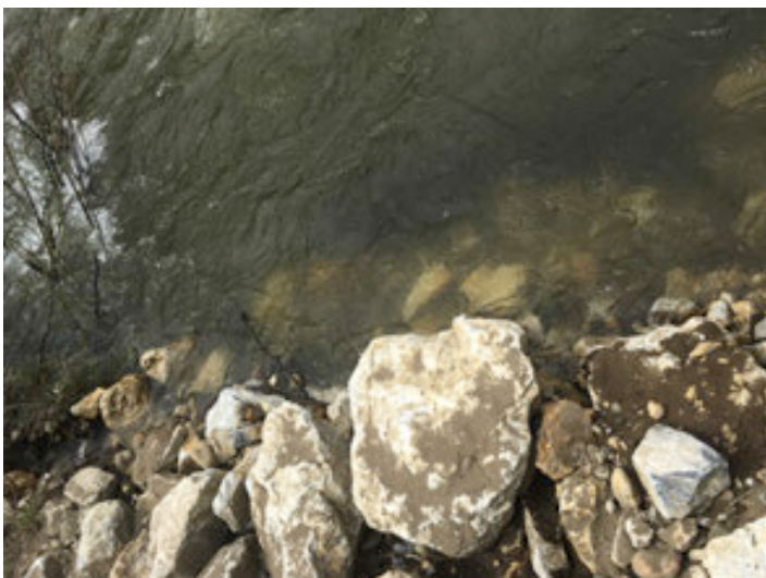
PHOTO 48: Launching riprap toe.
