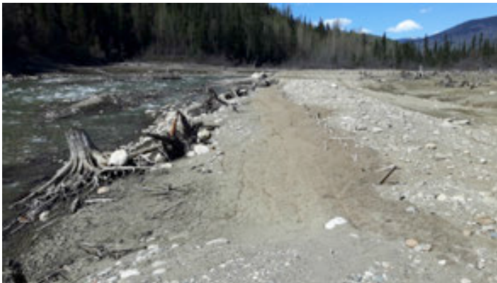
PHOTO 28: Coir Soil Wraps in Good Condition
