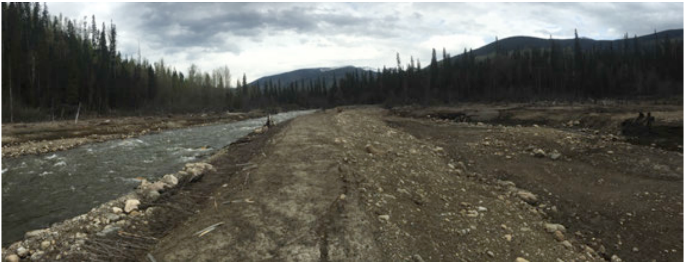
PHOTO 31 (Panoramic): Berm 'C' looking upstream from downstream end.
