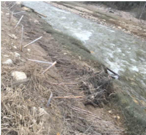
PHOTO 36: Coir soil wraps, willow brush layers along berm and native grasses/reeds at toe
