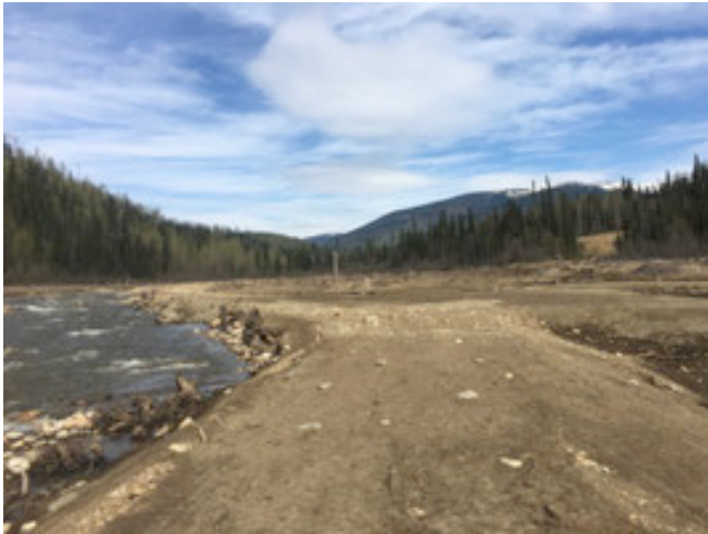
PHOTO 22: Looking Upstream at Berm 'D'
