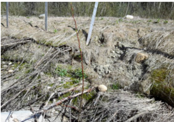
PHOTO 54: Moose related damage on creek-side slope (mostly to ECM layer)
