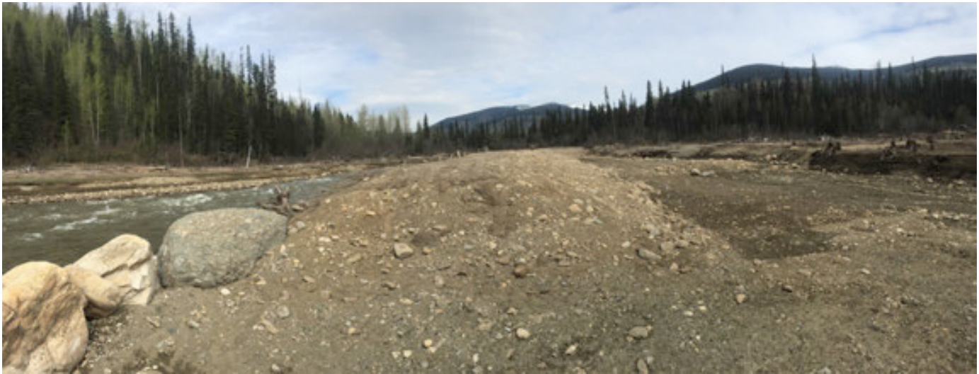
PHOTO 30 (Panoramic): Downstream end of Berm 'C' looking upstream.
