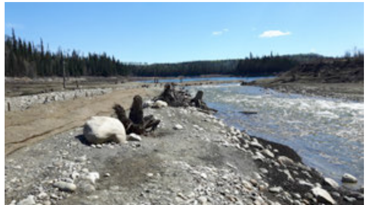
PHOTO 29: There Appears to be Some Deposition at the Berm Toe (and Channel Erosion in Thalweg)
