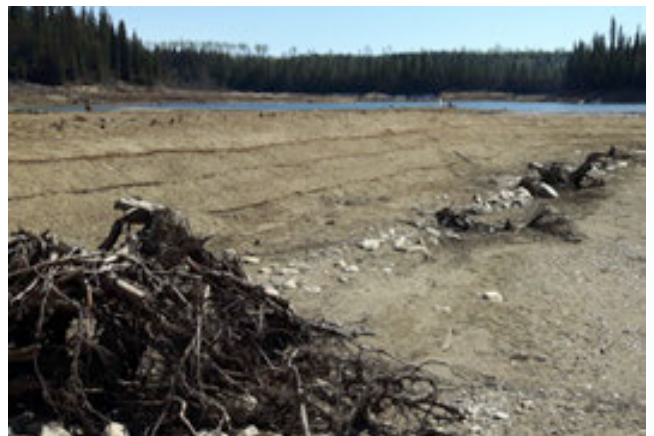
PHOTO 19: Coir Soil Wrap Layers in Good Condition. Note Upper Layer is ECM.
