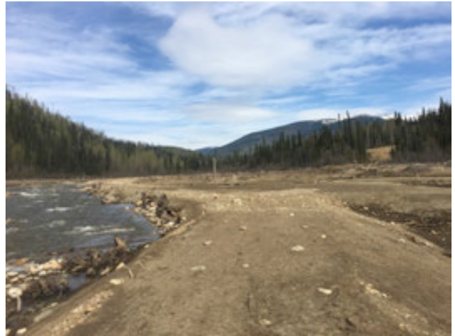
PHOTO 15: Upstream End of Berm 'F' Looking Upstream
