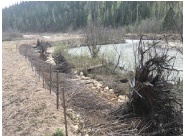
PHOTO 51: Soil wraps, willow brush layers, LWD and riprap looking downstream
