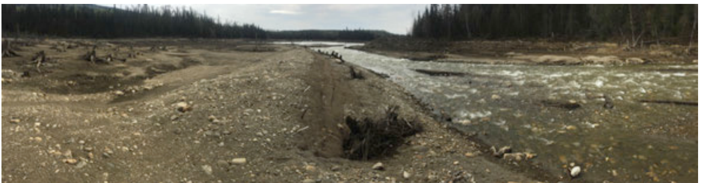
PHOTO 26 (Panoramic): Looking Downstream at Berm 'B'
