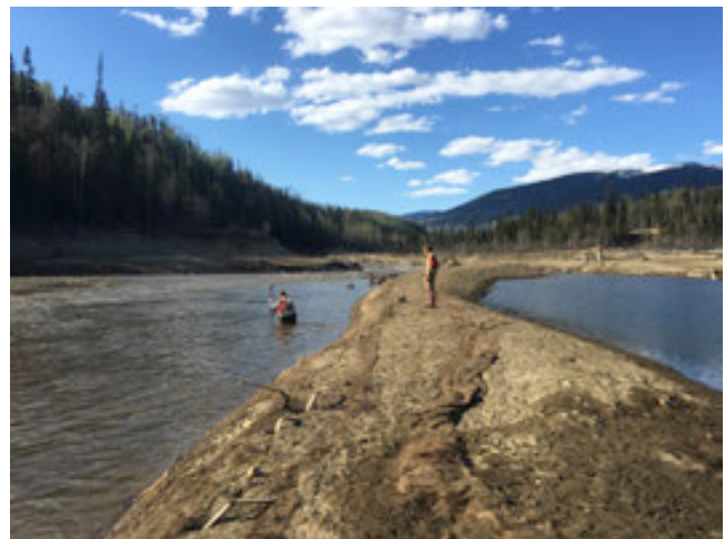
PHOTO 13: Berm 'F' Looking Upstream (Note Damaged/Decomposing ECM)
