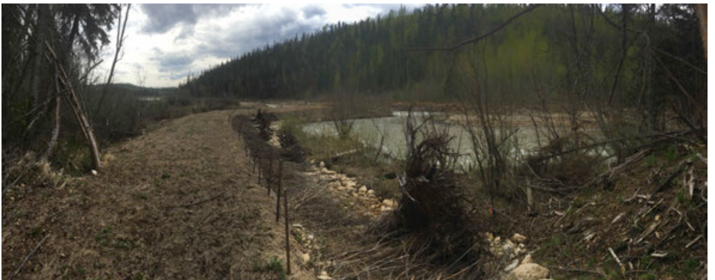
PHOTO 44 (Panoramic): Looking downstream at Berm 'J'
