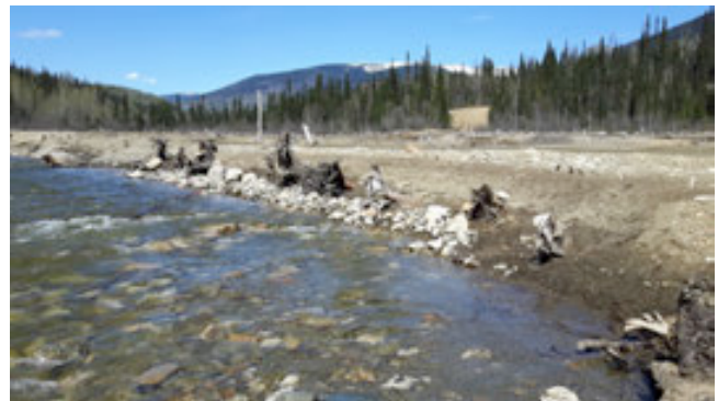
PHOTO 25: Deposition and Erosion Near LWD
