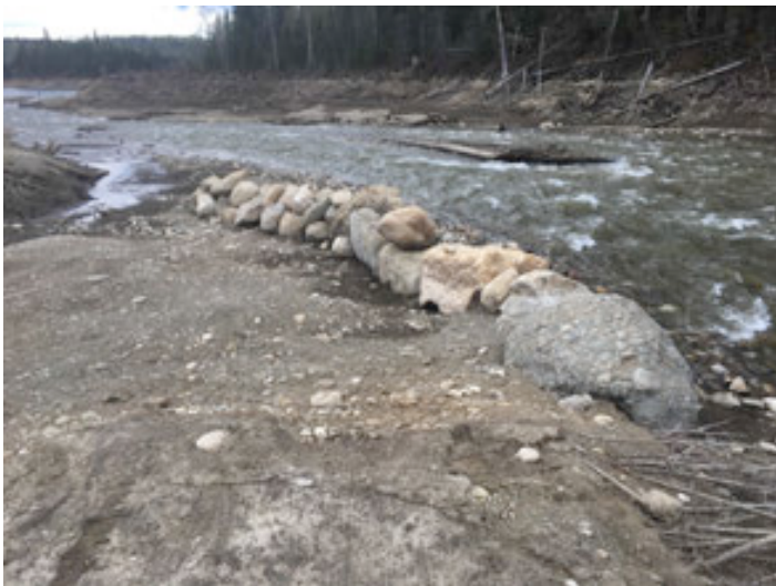
PHOTO 34: Downstream end of Berm 'C' looking downstream
