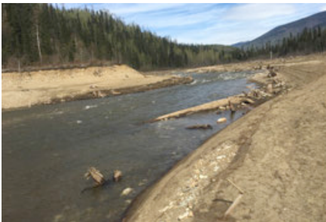
PHOTO 18: Deposited Log Along LWD and Deteriorating ECM
