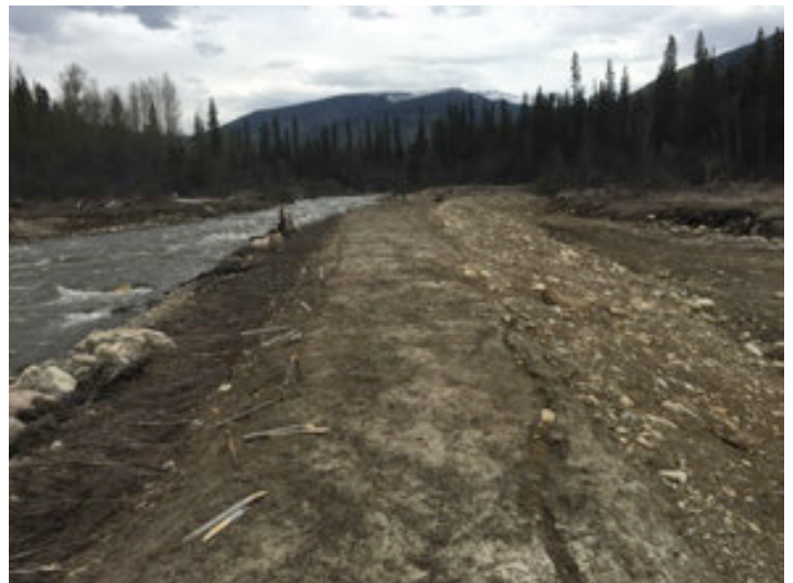
PHOTO 35: Downstream end of Berm 'C' looking upstream
