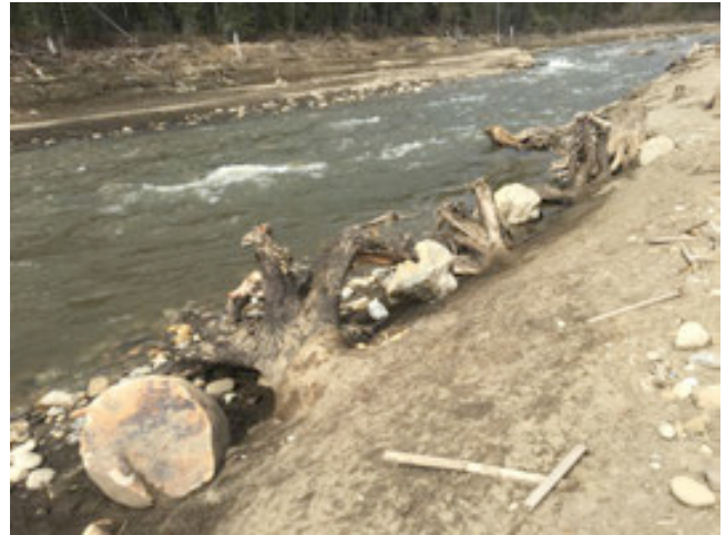
PHOTO 23: LWD at Berm 'D'.
