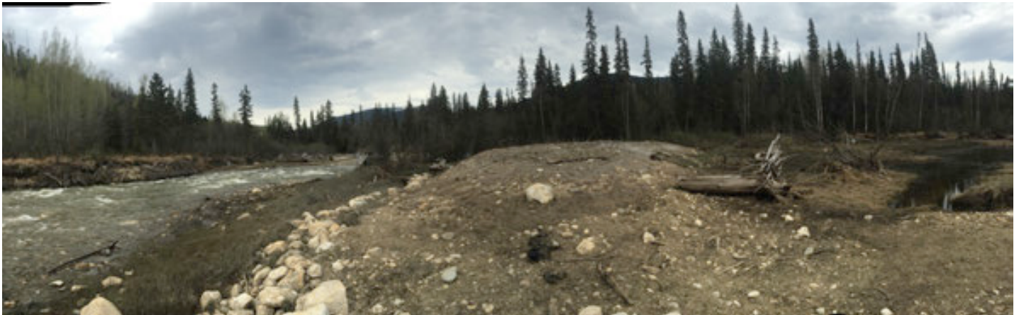
PHOTO 42 (Panoramic): Downstream end of Berm 'J' looking upstream. (Note black geotextile in foreground which is likely silt fence material, not bulk bag material, which is white.)
