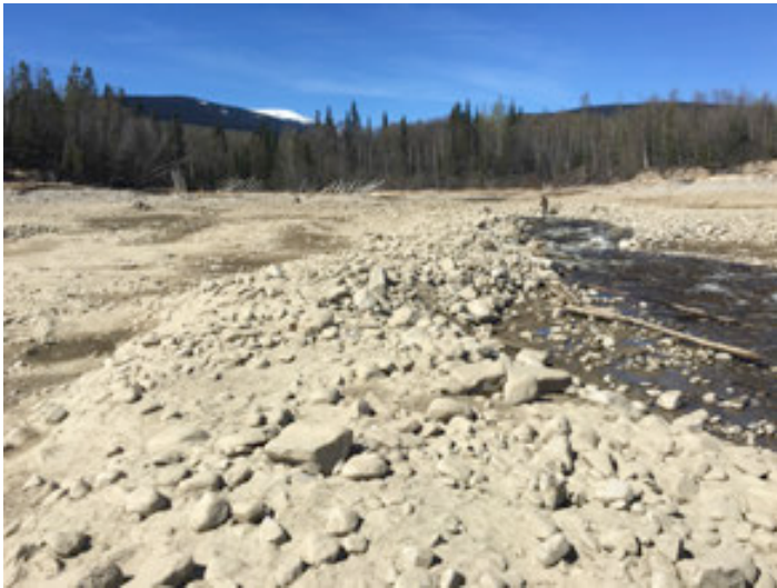
PHOTO 27: Looking upstream at lower Berm 'C' from downstream end of berm. Note uneven top of berm, some large cobble proud of crest.
