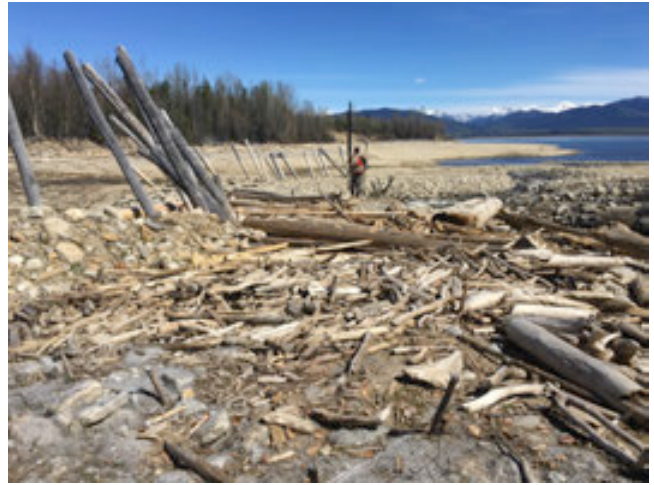
PHOTO 37: Flotsam at downstream end of Berm 'A' looking downstream
