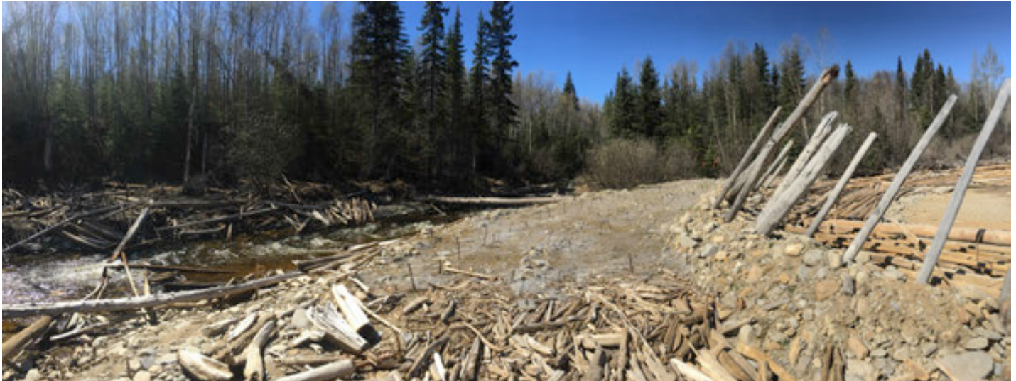
PHOTO 33 (Panoramic): Downstream end of Berm 'A' (note flotsam) and woody debris catcher
