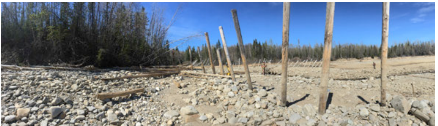
PHOTO 24 (Panoramic): Looking upstream at Berm 'C' and woody debris catcher
