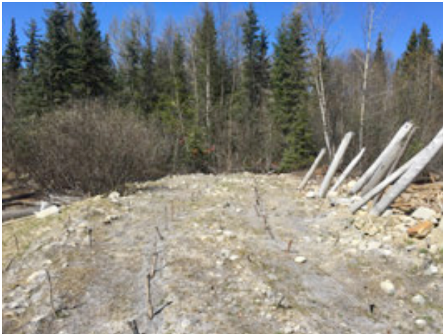
PHOTO 38: Upstream end of Berm 'A'
