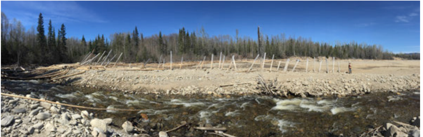
PHOTO 31 (Panoramic): Berm 'A' and left bank woody debris catcher
