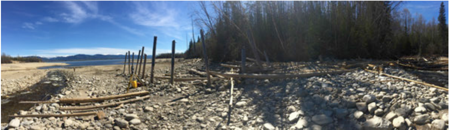
PHOTO 23 (Panoramic): Looking downstream at Berm 'C' and woody debris catcher
