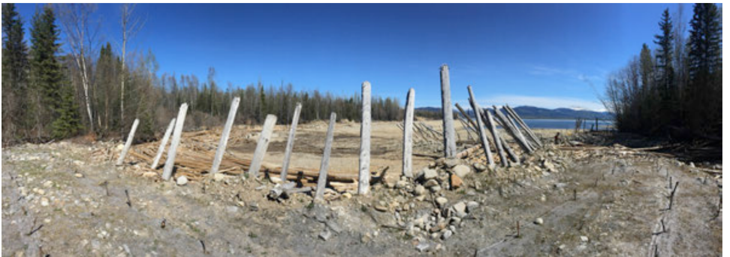
PHOTO 32 (Panoramic): Berm 'A' and left bank woody debris catcher (note bend is exaggerated)
