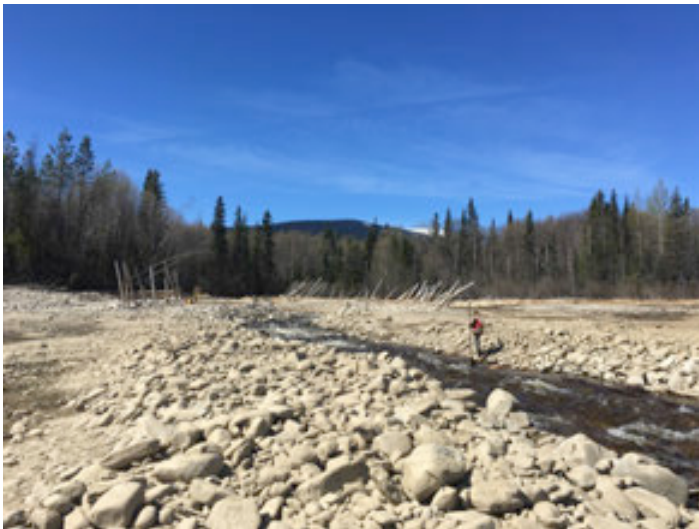
PHOTO 29: Looking upstream at Berm 'C' from downstream end of berm.
