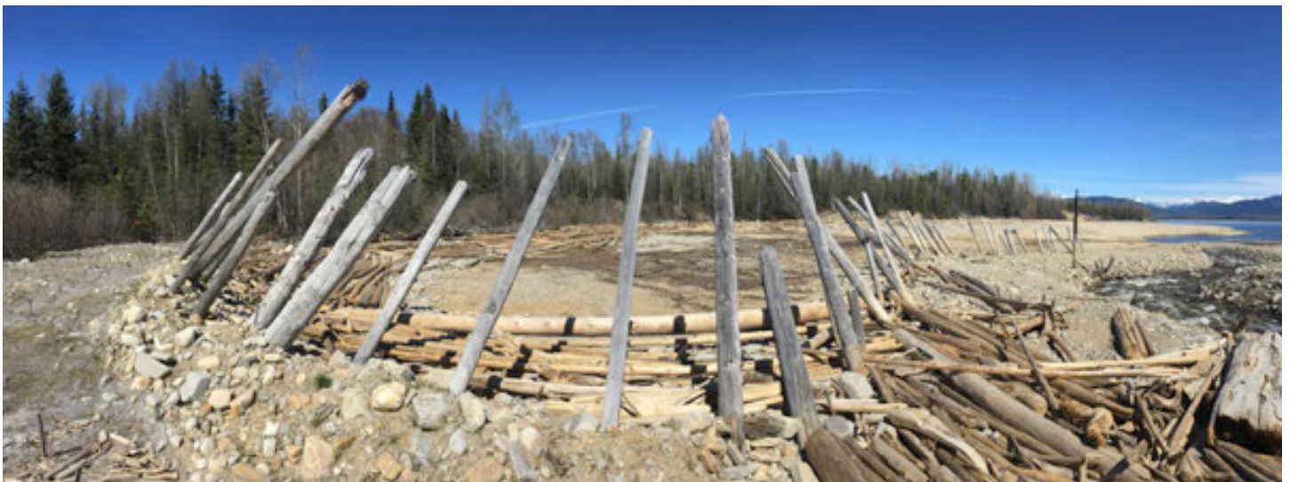
PHOTO 34 (Panoramic): Woody debris catcher with captured wood visible behind the upright logs. Some wood debris not captured is visible to the right (note bend is exaggerated in panoramic).
