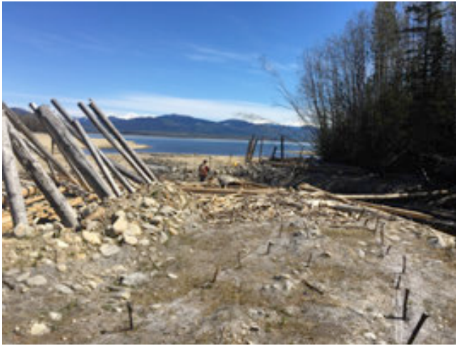
PHOTO 36: Downstream end of Berm 'A' looking downstream
