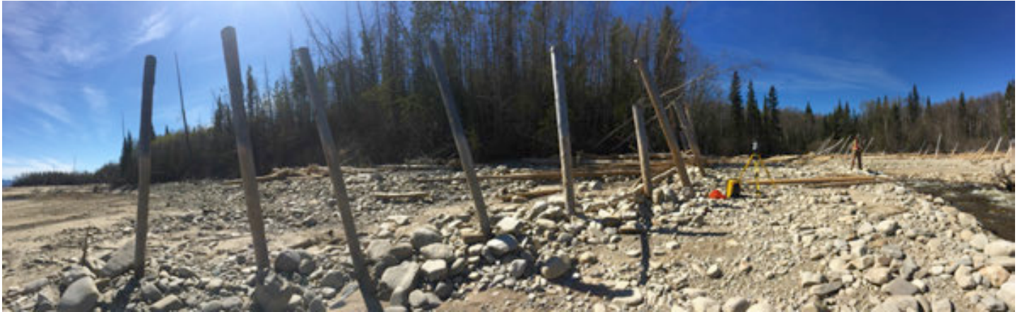
PHOTO 21 (Panoramic): Looking upstream at Berm 'C' and woody debris catcher
