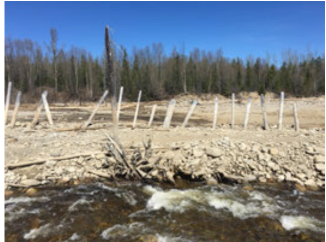
Photo 43: Embedded LWD in Berm 'A'
