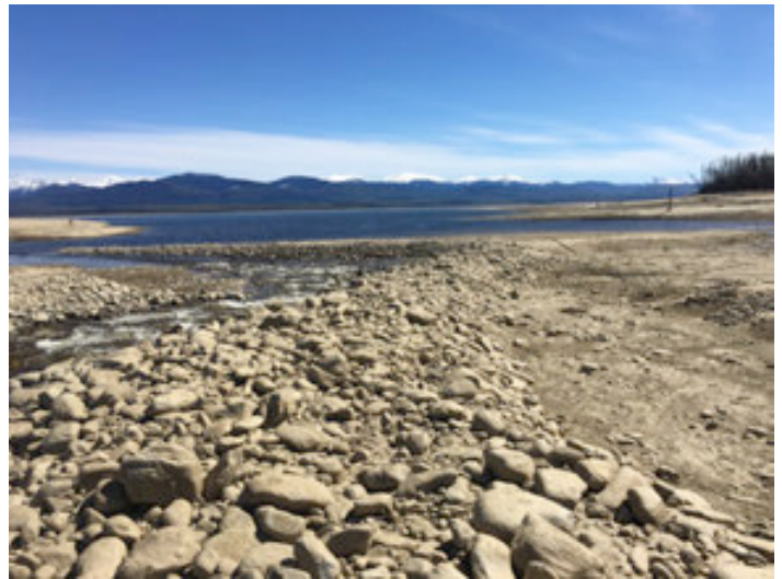
PHOTO 28: Looking downstream at Berm 'C'. Armour layer of cobble in good condition.
