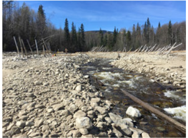
PHOTO 48: Looking upstream opening between left and right bank woody debris catchers
