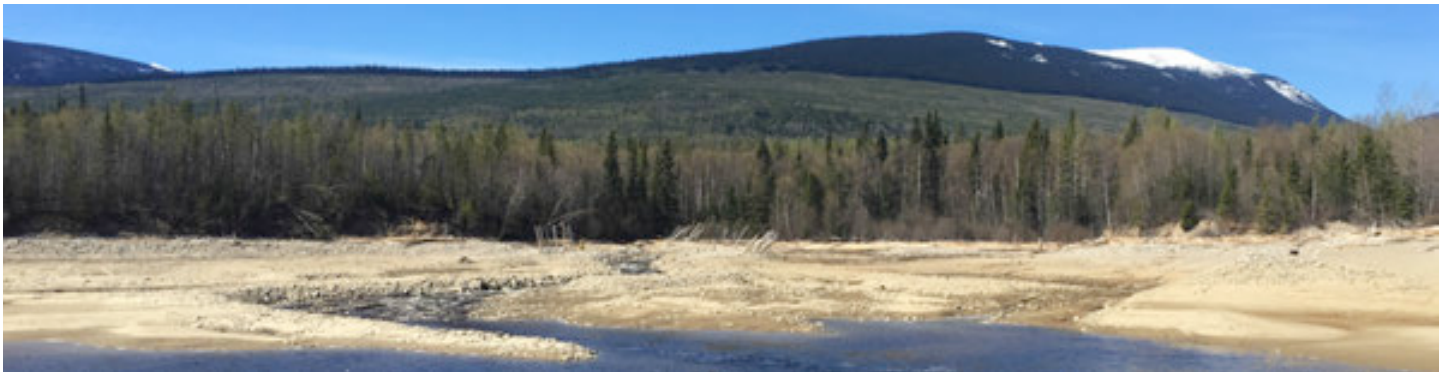
PHOTO 2 (Panoramic): Ole Creek works looking upstream from downstream left bank
