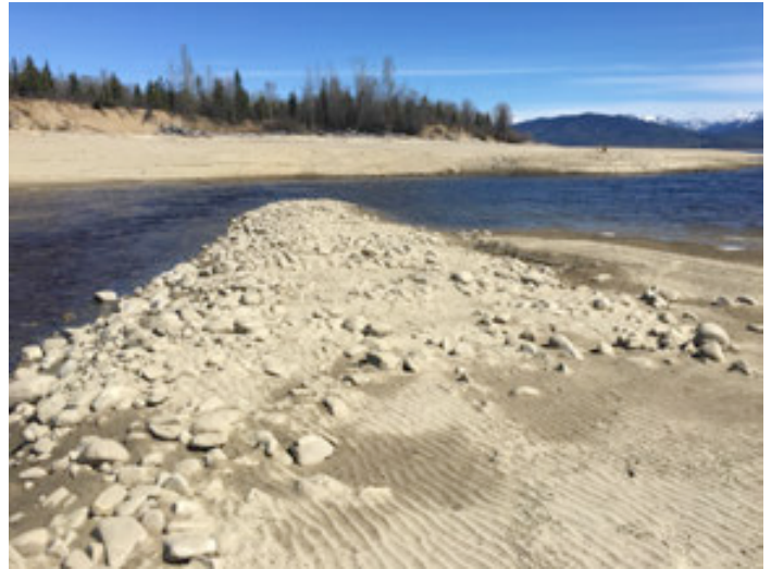
PHOTO 9: Berm 'D' looking downstream
