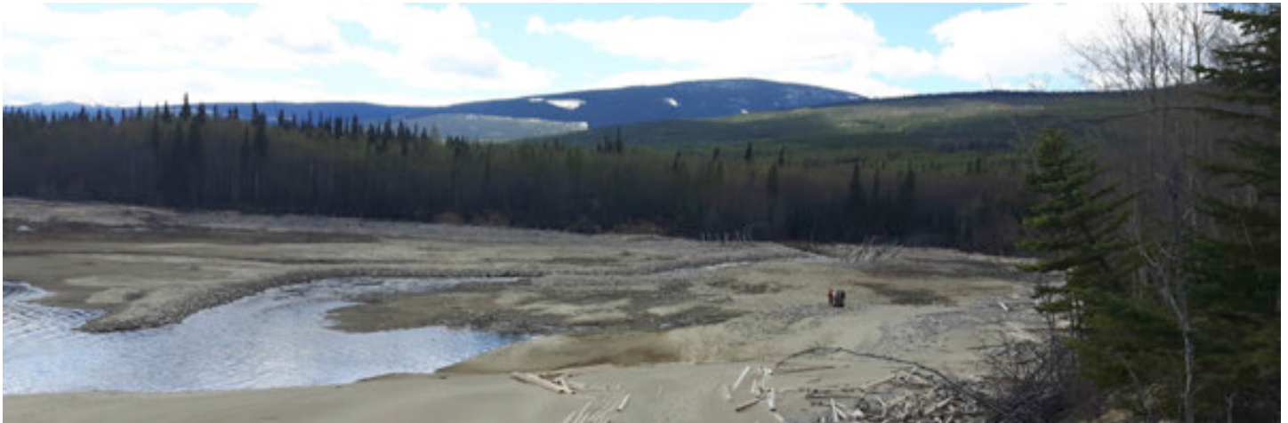
PHOTO 1 (Panoramic): Ole Creek works looking upstream from downstream left bank
