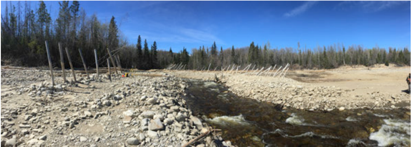
PHOTO 22 (Panoramic): Looking upstream along Berm 'C' and woody debris catcher (on left in photo)
