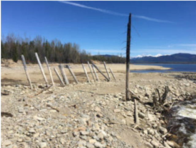
Photo 42: Downstream end of Berm 'A' and LWD embedded in berm (left side of photo)
