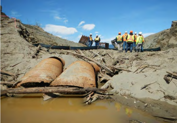
Photo 1 – Excavation & removal of old culverts.
