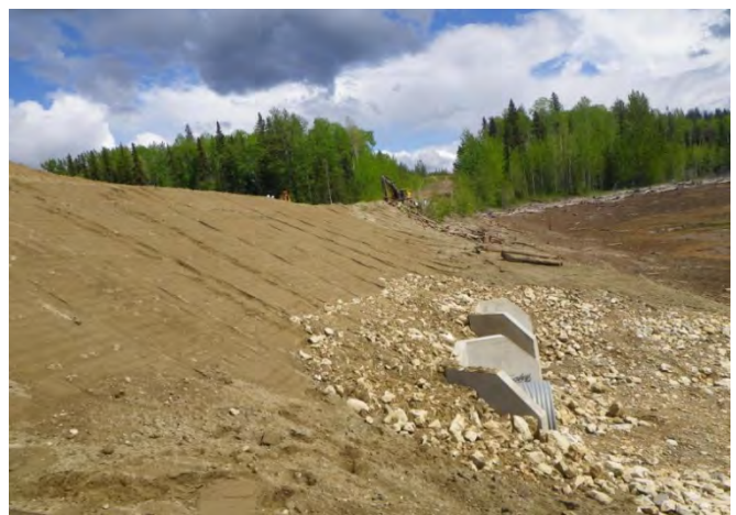
Photo 20 – Fill placement & view of headwalls, reservoir.
