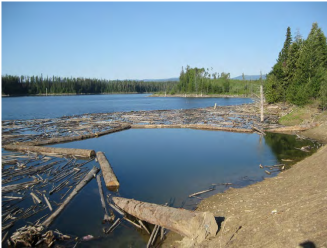
Photo 23 – Log boom installed south side, reservoir.
