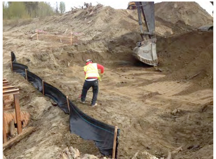
Installing silt fence
