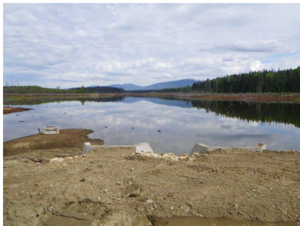
Upstream during construction
