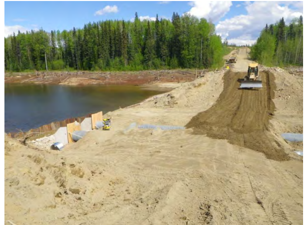
Culvert construction progress to top of culverts
