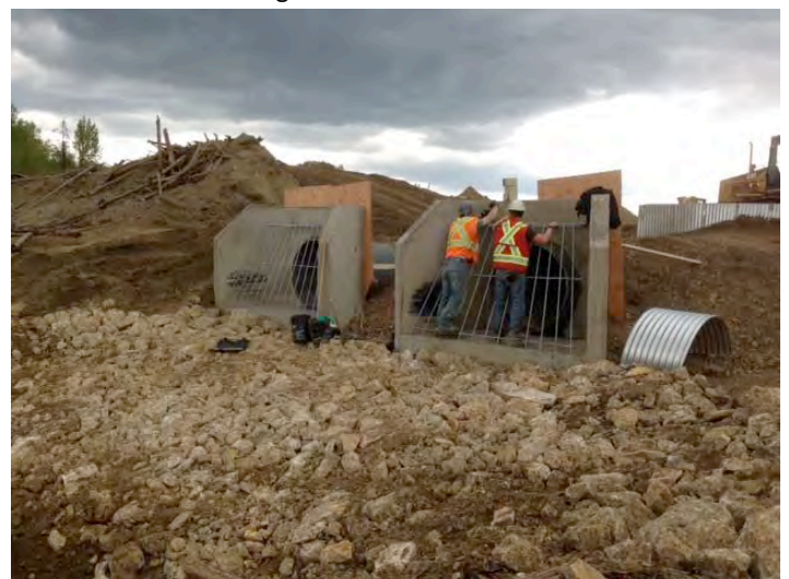
Installing Galvanized Grillage
