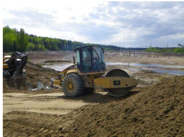
Compaction progress, road above culverts
