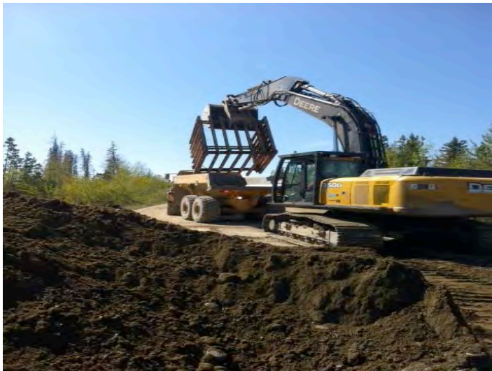
Loading out steel grates
