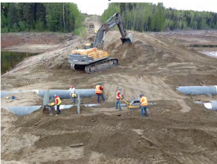
Backfilling culvert
