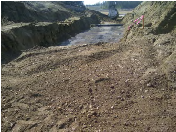
Placing Geo-grid and soil, upstream
