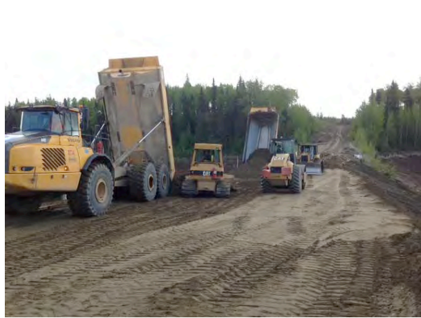
Spreading and compacting lifts
