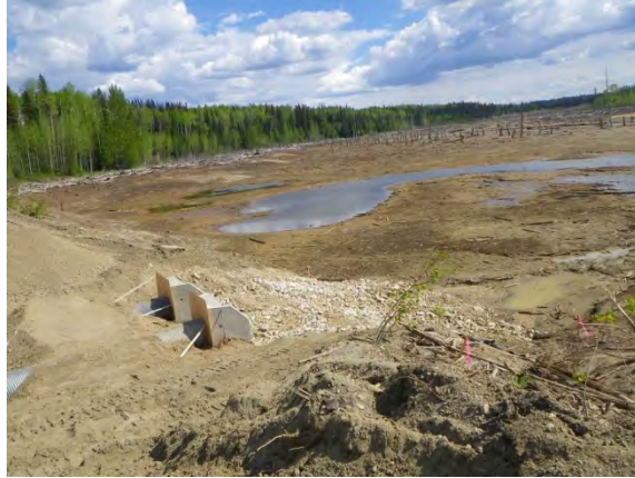
Culverts against concrete heads, downstream
