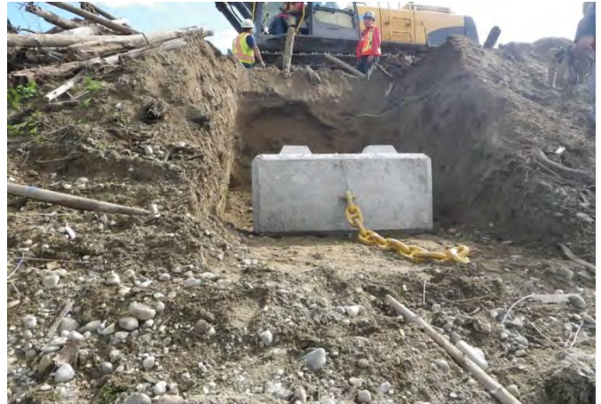
Photo 22 – Embankment anchor & 37.5 mm chain.
