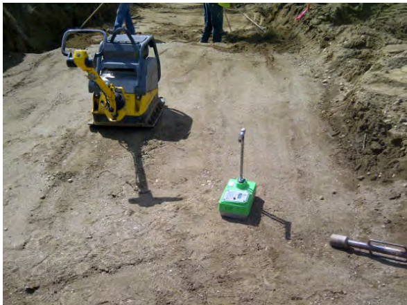
Testing density for 1 st layer above Geo-grid
