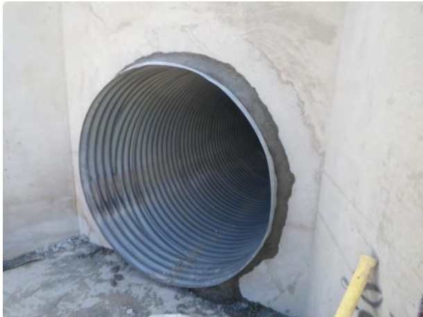
Culverts with grout against concrete heads, downstream
