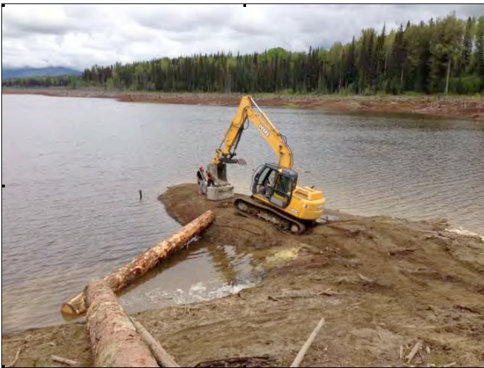
Placing upstream log boom
