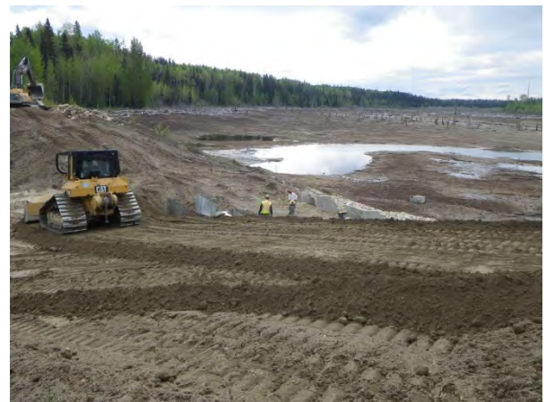
Downstream during construction
