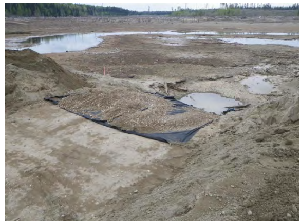
Placing Geo-textile, downstream.
