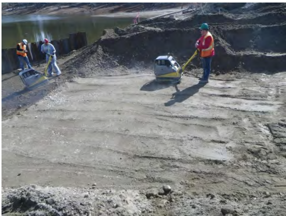
Progressing compaction, upstream
