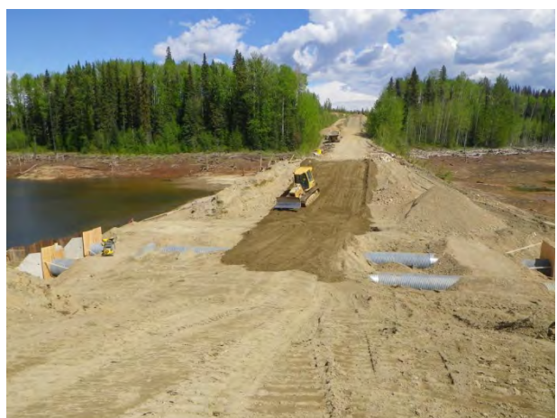
Culverts with grout against concrete heads, downstream
