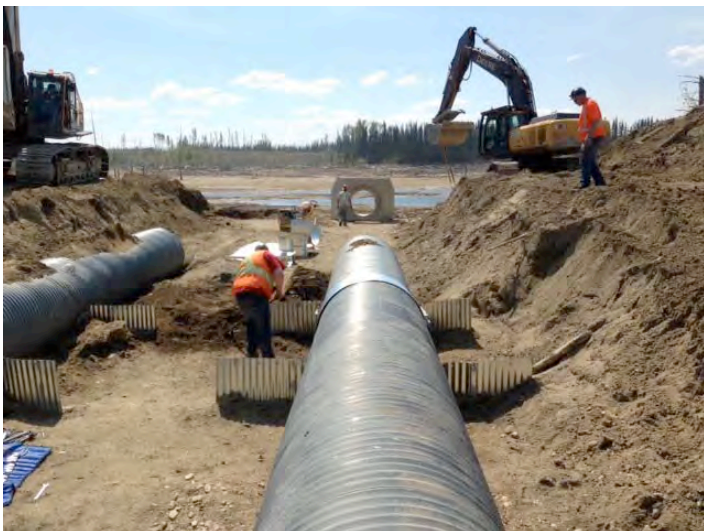
Placing culverts
