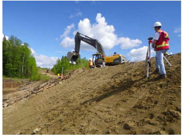
Slopes close to finishing, downstream
