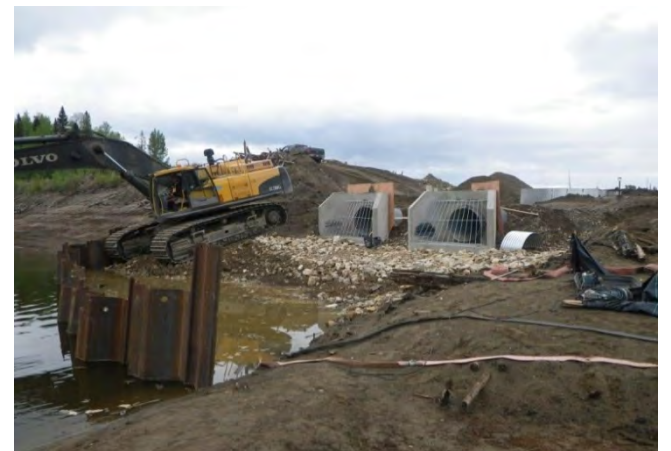
Photo 16 – Grillage installation on upstream headwalls.
