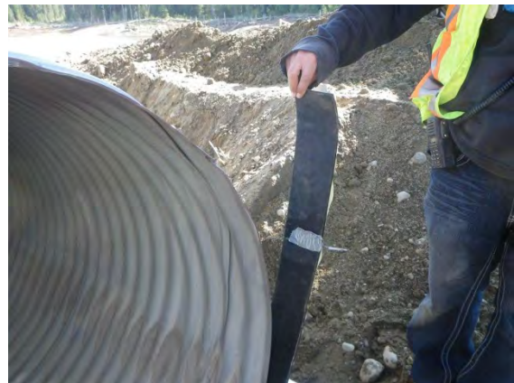
Seals for tying culvert pieces together
