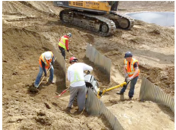
Backfilling final anti-seepage collar
