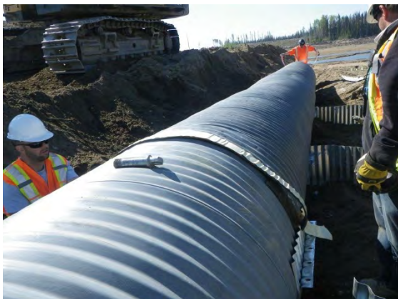
Tying culvert pieces together
