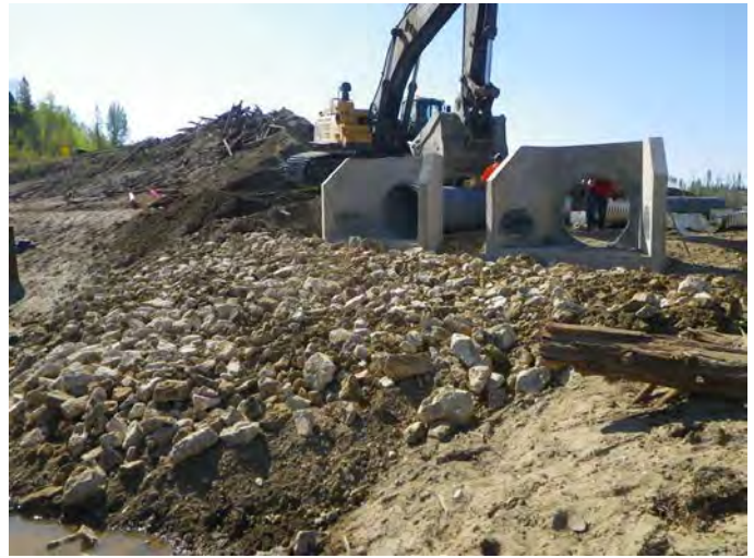
Photo 6 – Placement of Class 10 kg riprap.
