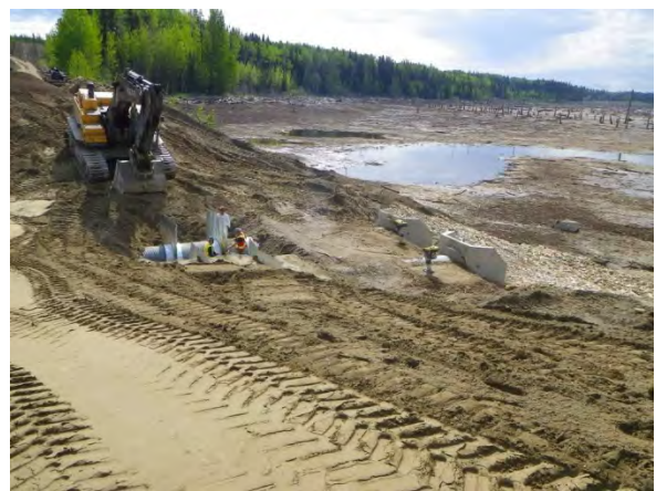
Compaction progress, road above culverts
