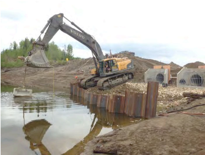
Placing Anchor Blocks
