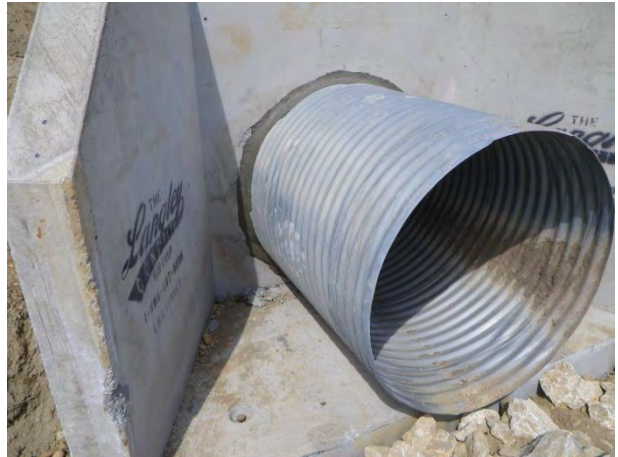
Culverts with grout against concrete heads, downstream
