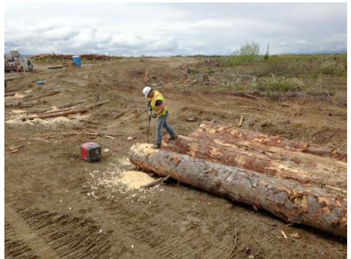
Drilling boom chain holes
