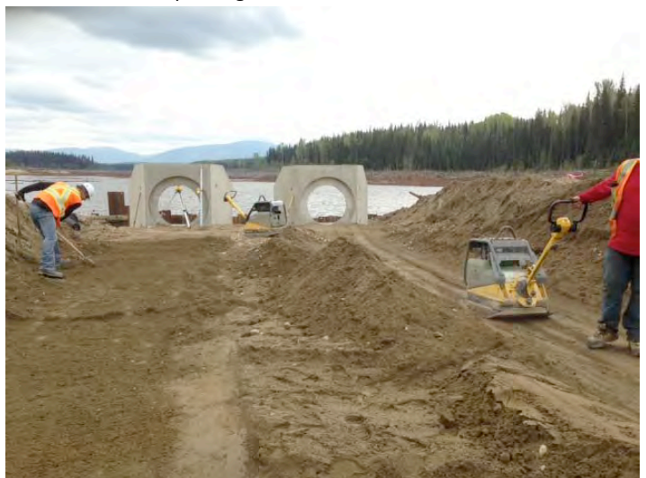
Headwalls on the inlet
