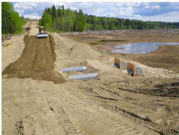
Culvert construction progress showing downstream and upstream
