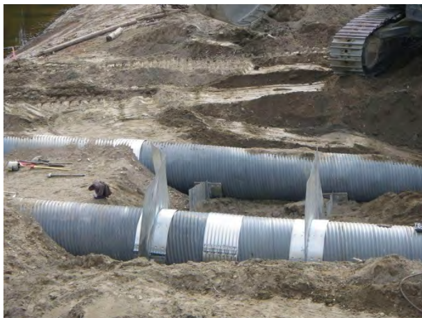
Culvert construction progress to top of culverts
