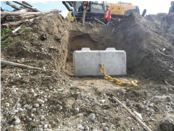
Placing concrete blocks embedded in slopes
