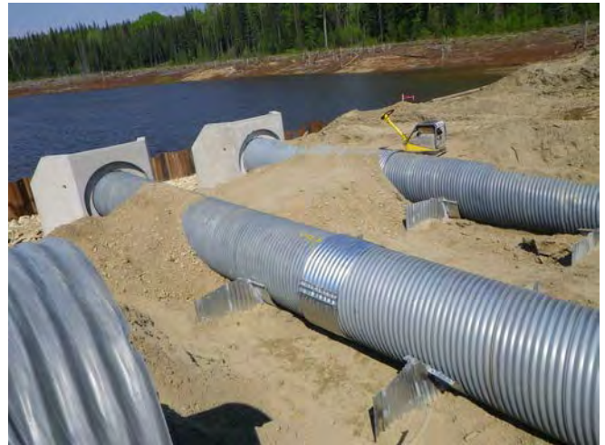
Photo 10 – Twin culvert installation.
