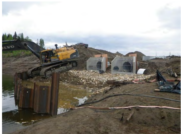
Placing concrete blocks for anchors, upstream.
