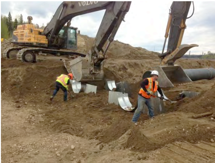
Installing anti-seepage collars
