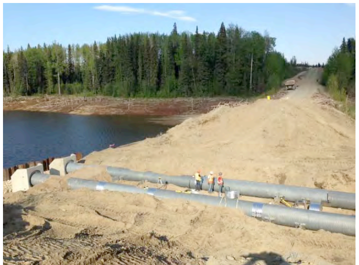
Culverts in place
