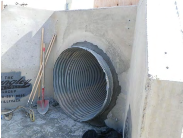
Culverts with grout against concrete heads, upstream
