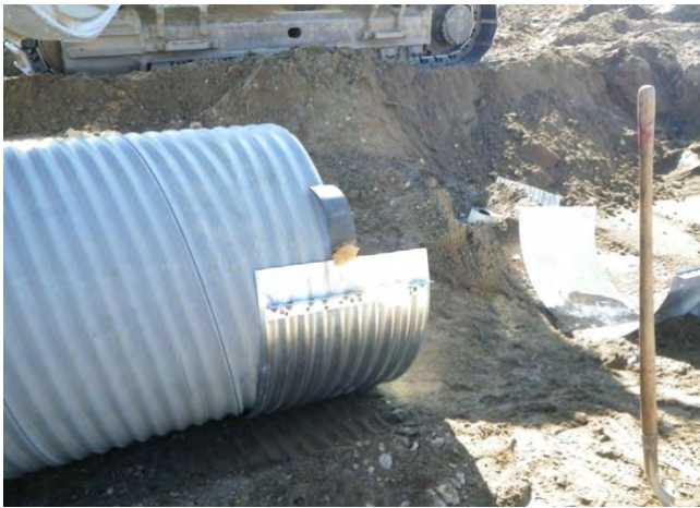
Photo 7 – Culvert couplings and neoprene gaskets.
