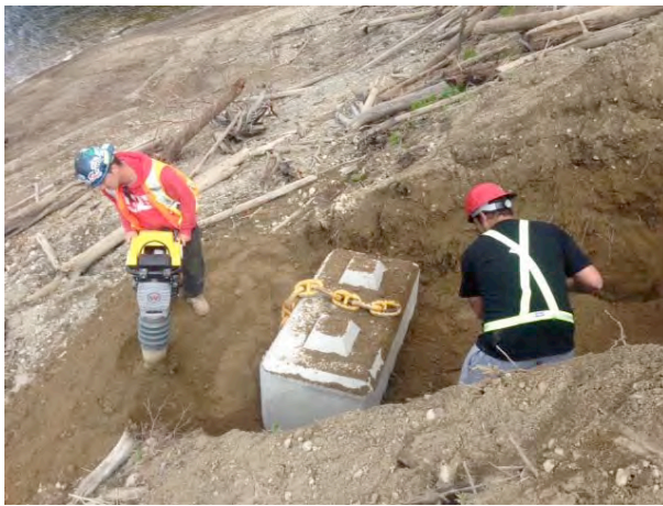
Backfilling embankment anchors
