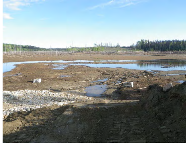
Photo 18 – Log boom anchor block placement reservoir.
