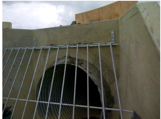
Erecting steel guards against concrete heads
