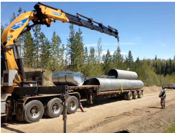
Offloading culverts
