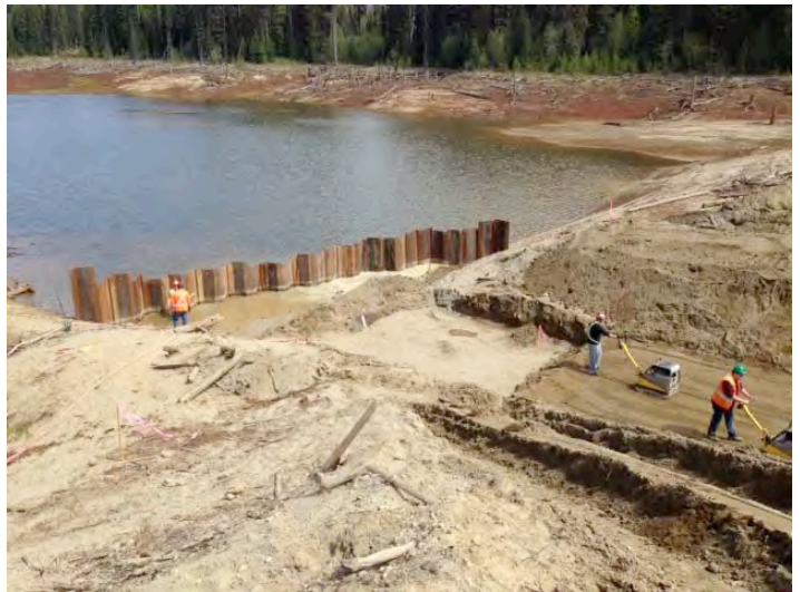
Compacting the culvert beds
