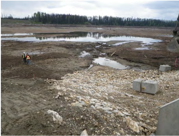
Placed concrete blocks downstream
