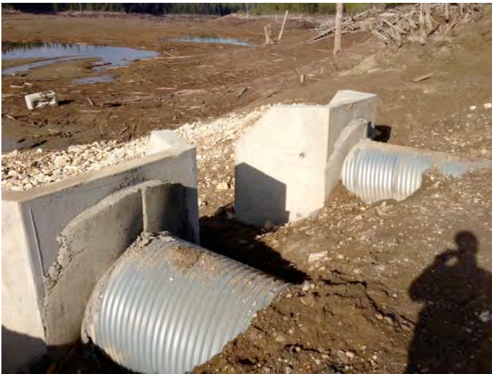
Concrete around culverts
