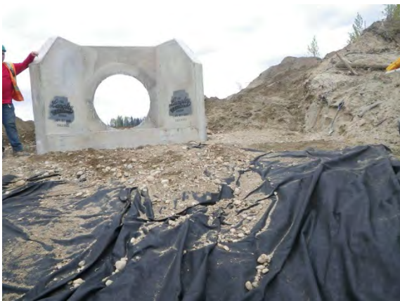
Placing Culvert Concrete Head
