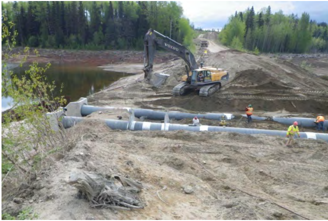
Photo 13 – Culvert installation – north side – lagoon.
