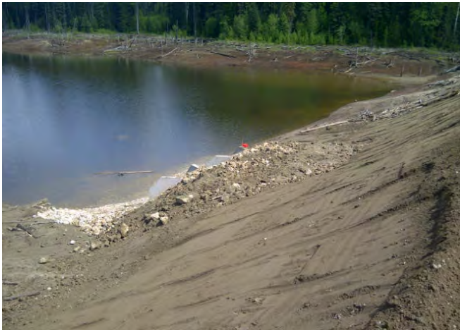
Photo 19 – Fill placement & view of headwalls, Lagoon.
