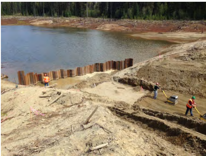
Levelling and packing lifts
