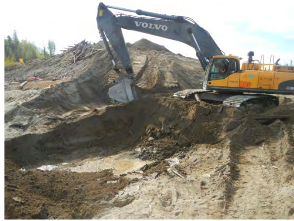
Excavating debris for Culvert base pre.
