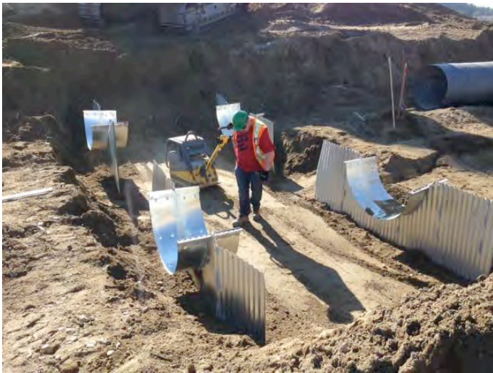
Compacting around anti-seepage collars
