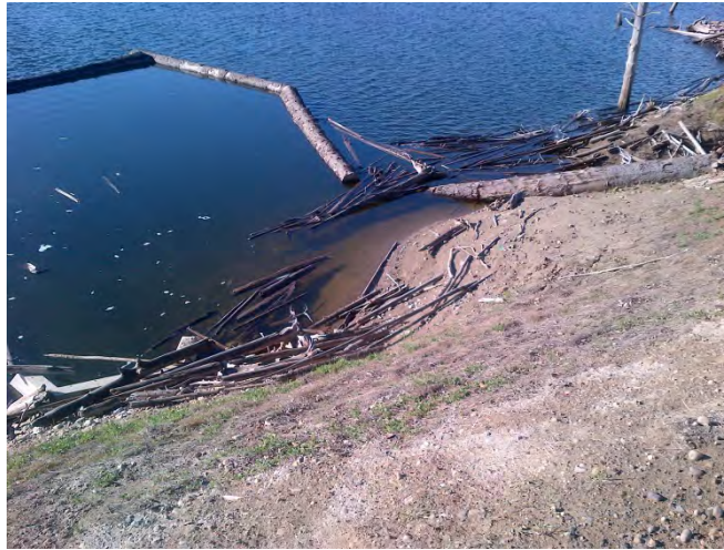
Photo 1 – October 2013 Post Construction Inspection – Logs bypassing log boom on reservoir side.
