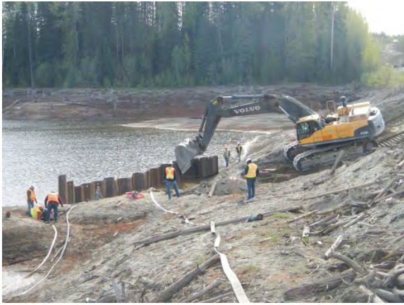
Building Sheet Pile Wall
