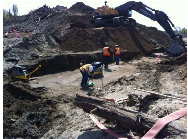
Geo Tech testing densities
