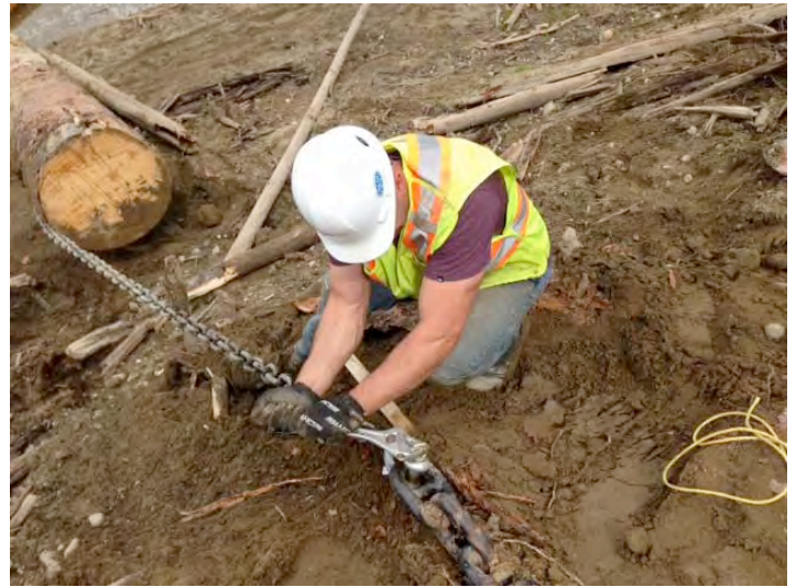
Fastening log boom to embankment block
