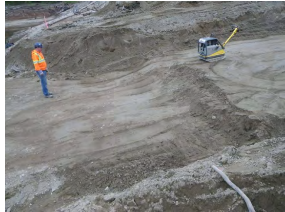
Progressing compaction mid-section
