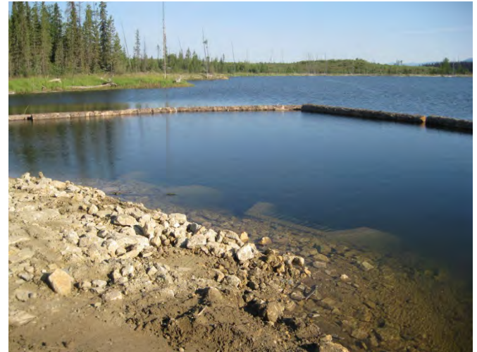
Photo 24 – Log boom installed north side, Lagoon.
