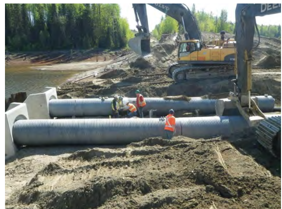
Tying culvert pieces together
