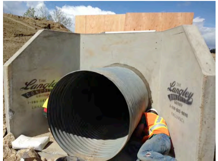
Grouting head walls
