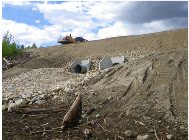
Placing concrete blocks embedded in slopes
