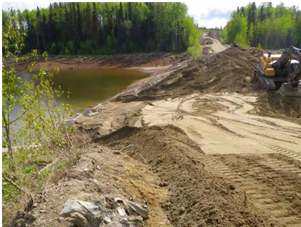
Compaction progress, road above culverts
