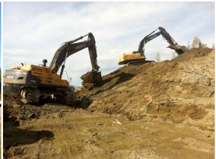
Safe sloping excavation
