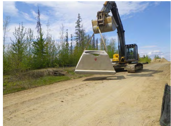
Transforming Culvert Concrete Head
