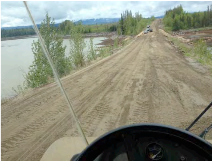
Grading and packing the Causeway
