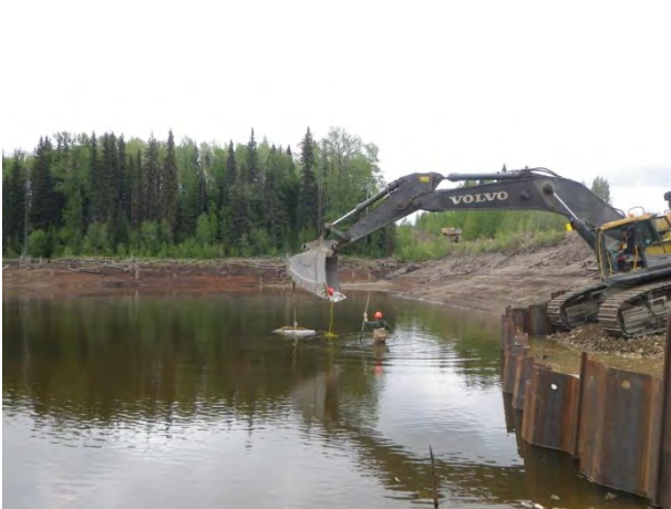
Placing concrete blocks for anchors, upstream.
