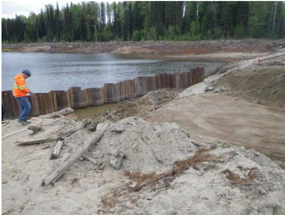
Progressing compaction, upstream
