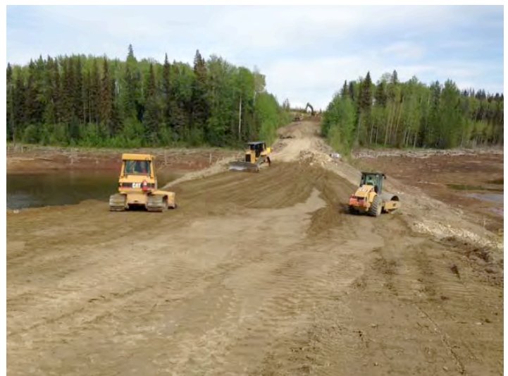
Spreading and compacting even lifts
