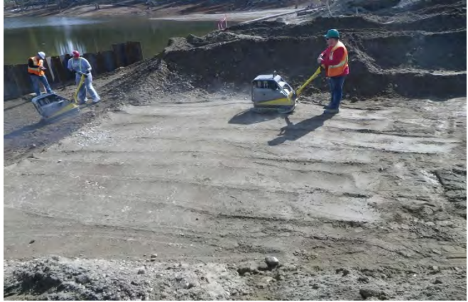
Photo 4 – Placement of fill material and compaction.
