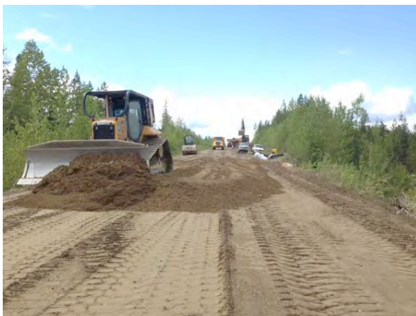
Spreading gravel base
