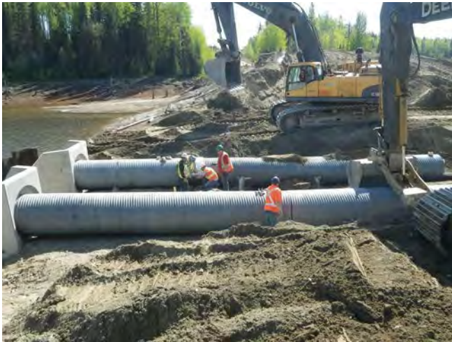
Photo - 9 Twin culvert installations.
