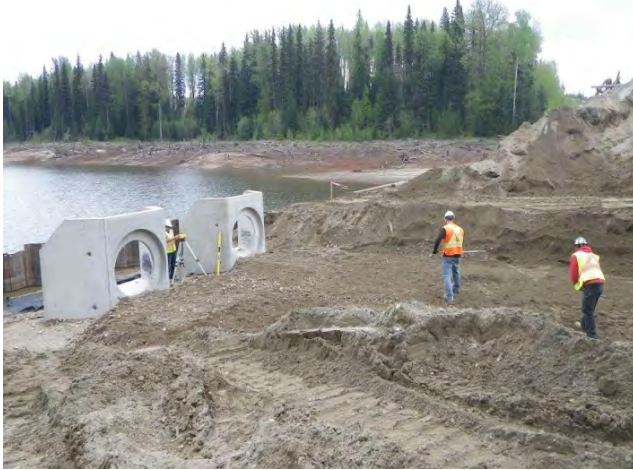
Photo 5 – Placement of culvert headwalls & geotextile.
