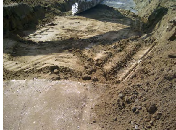
Culvert base excavation
