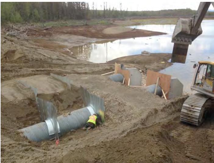
Installing Collars
