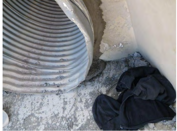
Culverts with grout against concrete heads, upstream
