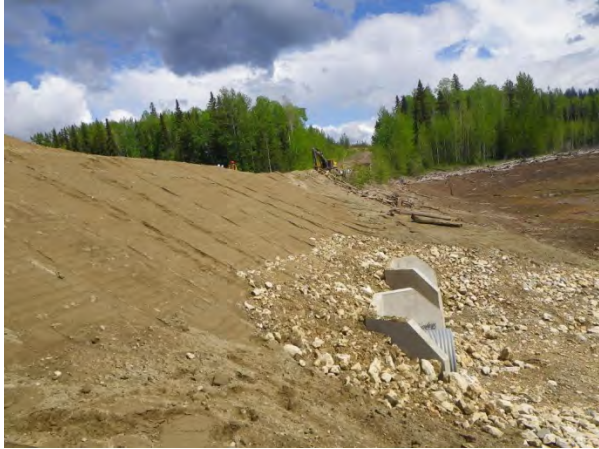
Slopes close to finishing, downstream
