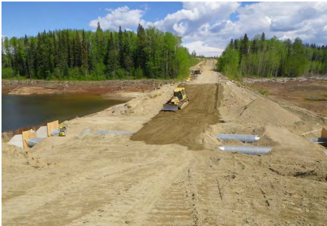
Photo 15 – Backfill around culverts and embankment.
