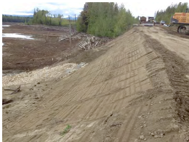
Slope on downstream side
