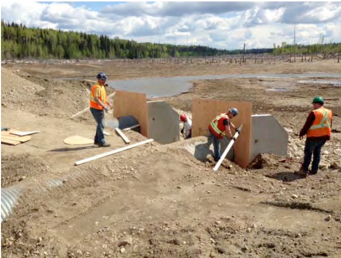
Framing head walls
