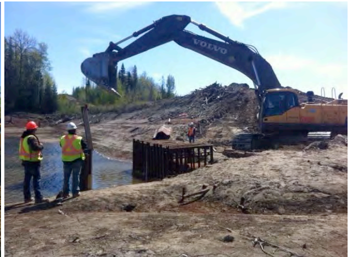
Installing coffer dam
