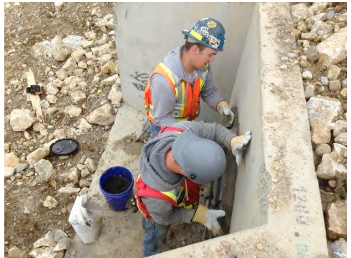
Re-grouting headwalls
