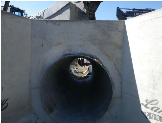
Erecting culvert against the concrete head
