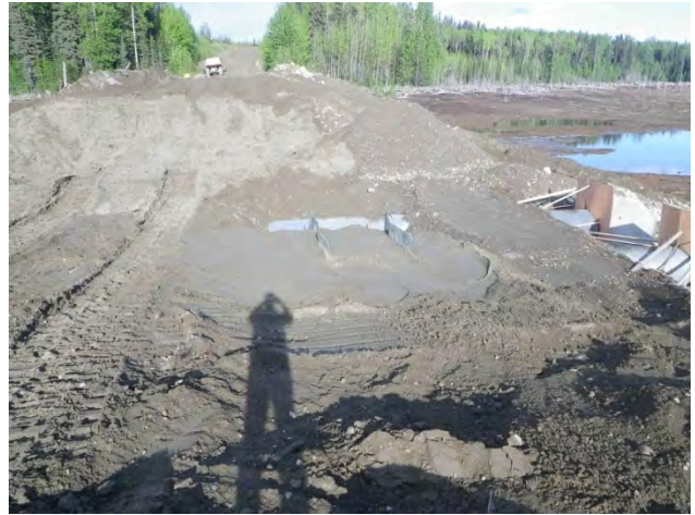
Compaction progress for road above culvert
