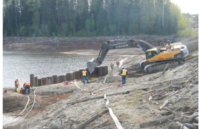
Photo 2 – Placement of sheet pile coffer dam.
