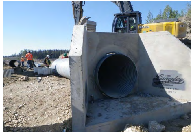
Photo 8 – Placement of anti-seepage collars.
