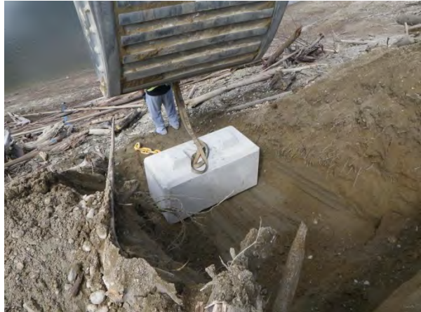
Placing concrete blocks embedded in slopes
