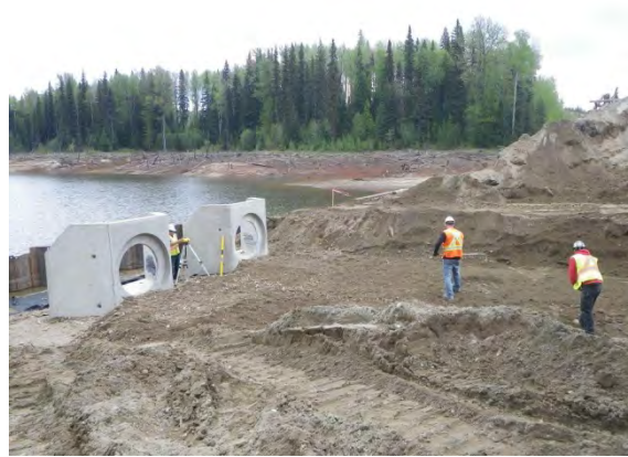
Prep. Culvert base, upstream
