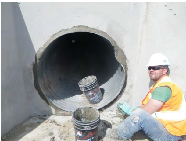
Culverts with grout against concrete heads, downstream
