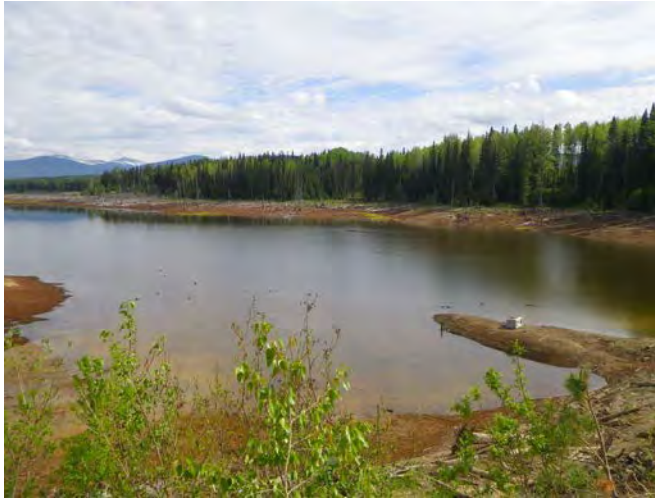
Photo 17 – Log boom anchor block placement lagoon.
