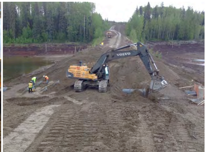
Backfilling Collars
