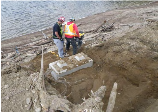
Photo 21 – Embankment anchor installation.
