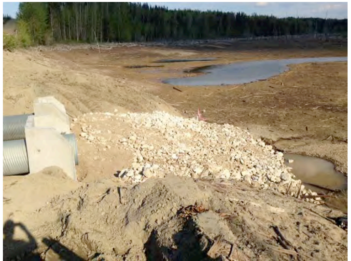
Installing rip-rap on downstream end
