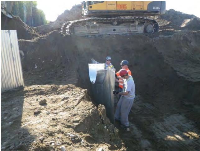
Photo 11 – Anti-seepage collar installation.
