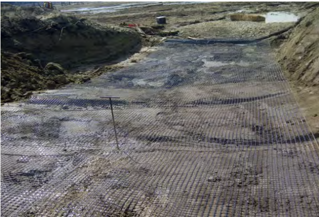
Photo 3 – Placement of geogrid.
