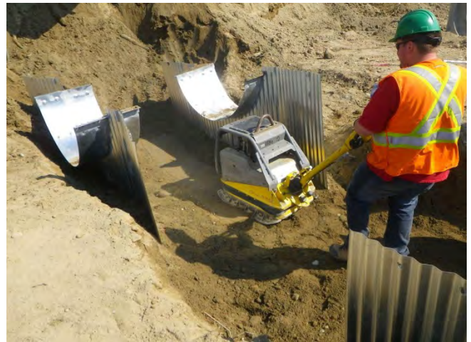
Photo 12 – Compaction.
