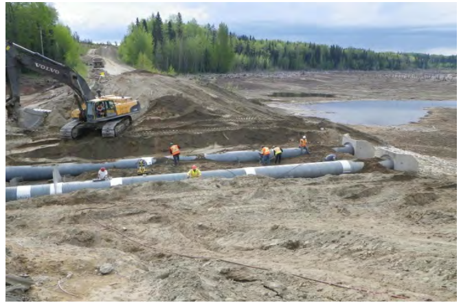
Photo 14 – Culvert installation, south side – Williston Reservoir.
