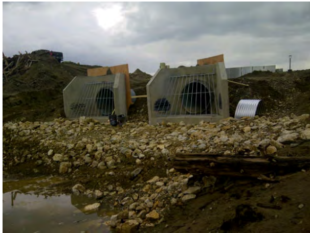
Erecting steel guards against concrete heads
