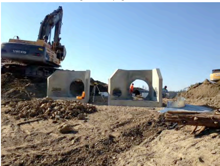
Headwalls on the inlet
