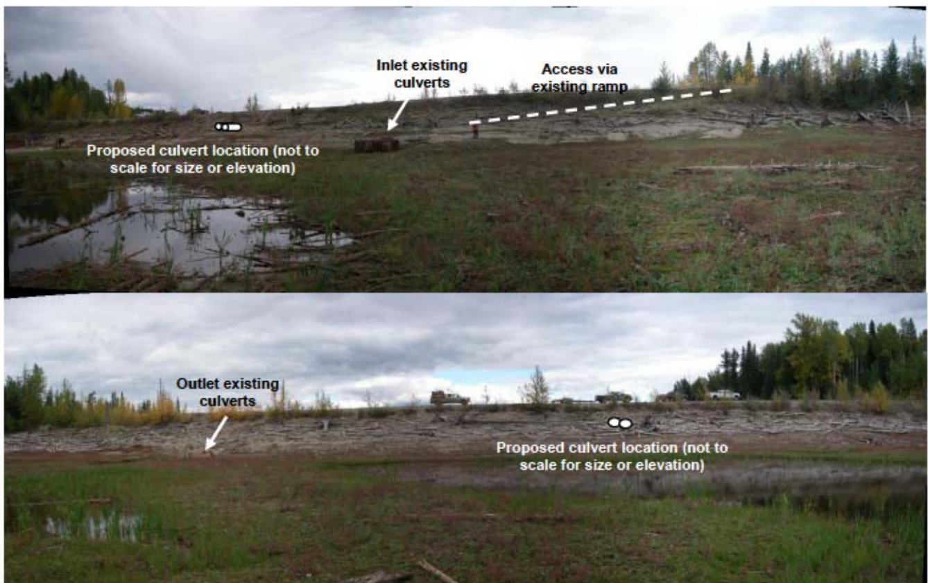
Photograph 13: Top - A view south (downstream) towards the causeway in September 2010, showing locations of existing features. The top of the cage is approximately 666.5 masl. Bottom - a view north (upstream) towards the downstream side of the causeway. Note the location of proposed new culverts is approximate and is not to scale for elevation or size. Design Drawing 1 in Appendix B provides these details.
