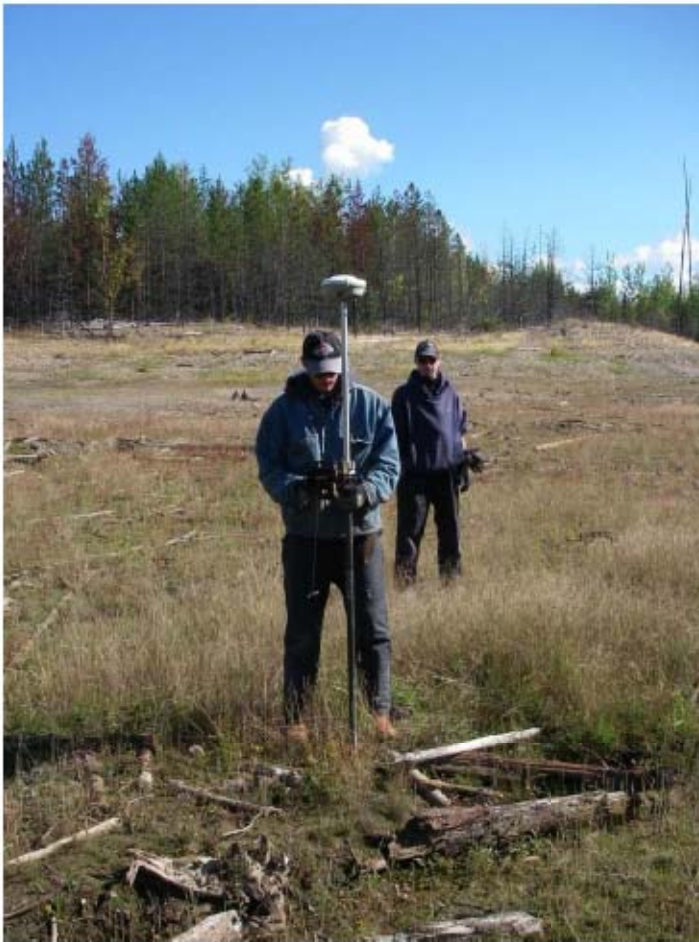
Photo 1: Surveyors from Vector completing topographic surveys of the basin at Site 34.
