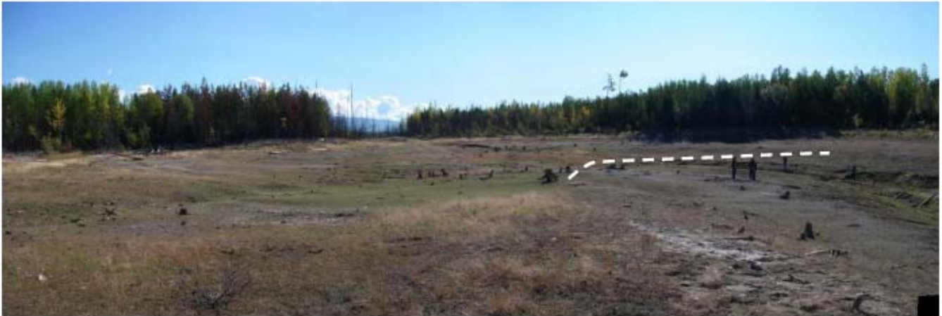
Photo 19: A view south east from the inlet towards the beaver pond. The white dotted line approximates the proposed positioning of the for the MacTubes™.
