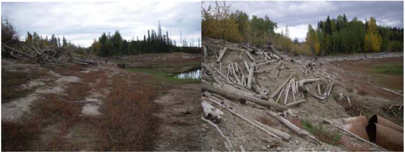
Photo 12: The base of the north (upstream) side of the causeway viewed west (left) and the base of the south (downstream) side of the causeway viewed east (right).
