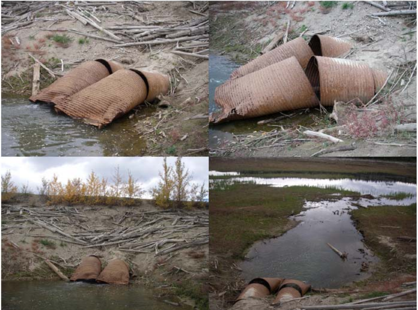
Photograph 8: Various views of the outlet of the two culverts on the south (downstream) side of the berm.
