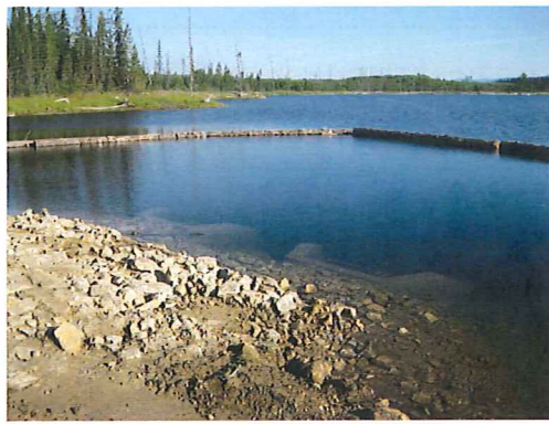
Airport Lagoon – Full Pool Post Construction
