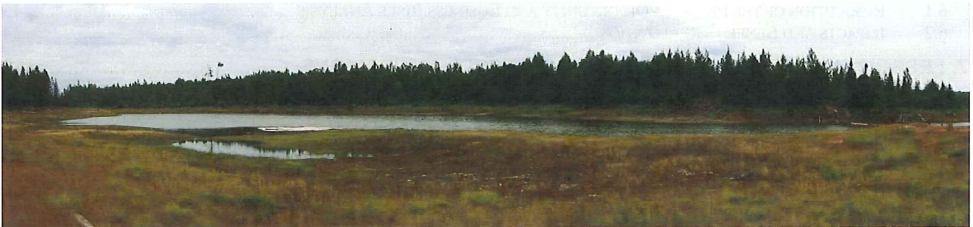
Beaver Pond – Full Pool Post Construction
