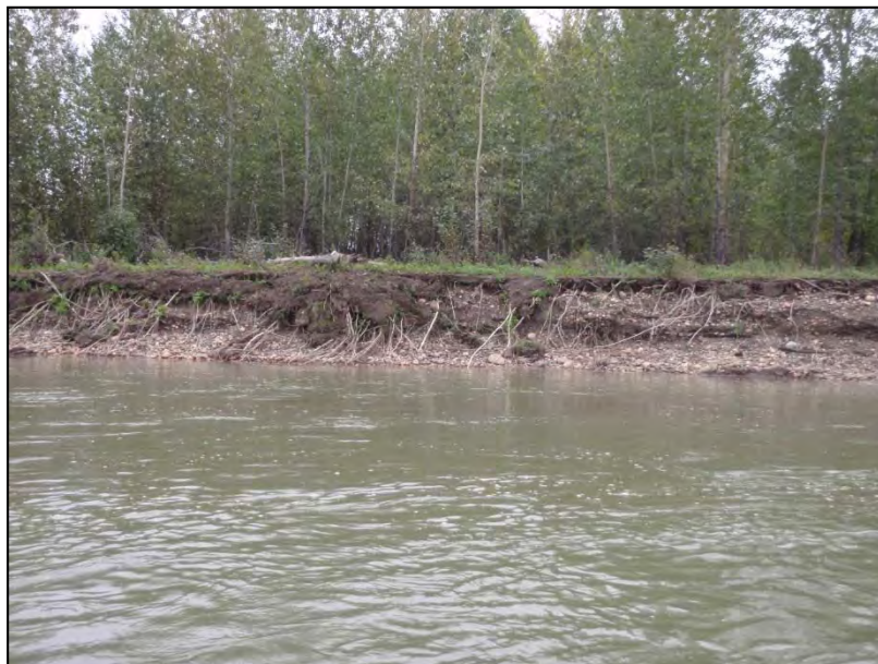
PHOTO 6 – Lower Pine River – typical site of active bank erosion.
