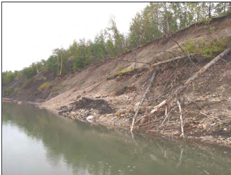
PHOTO 8 – Lower Pine River – typical glacio-fluvial bank materials.
