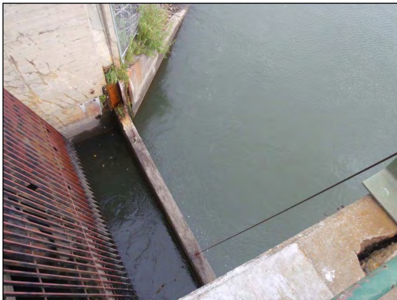
PHOTO 13 – Spectra Energy intake forebay.
