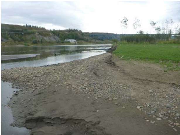
Photo 3-3 Erosion at NE corner of constructed 102.5R channel
