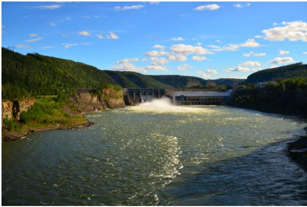
July 2012 spillway operations at Peace Canyon Dam
