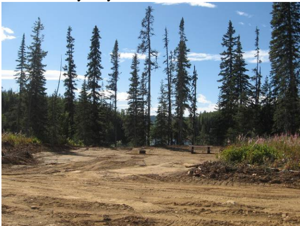
Six Mile Bay after upgrades August 18 2015
