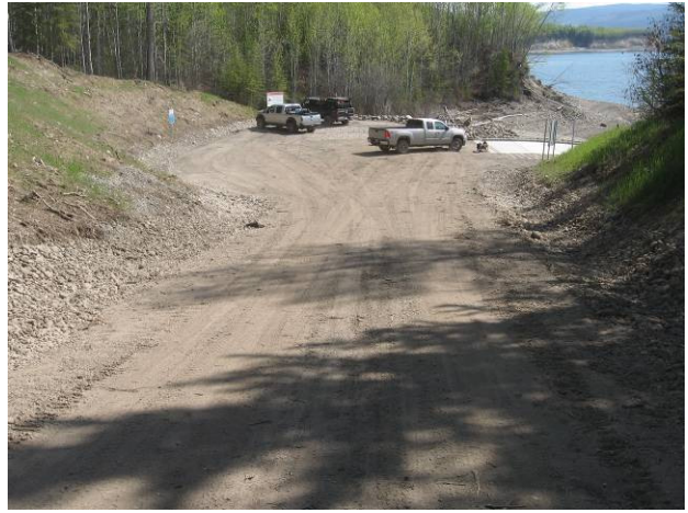
Dunlevy top of ramp May 15 2015
