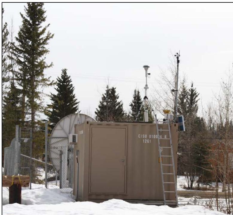
Figure 29: Kwadacha Air Quality Monitoring Station
