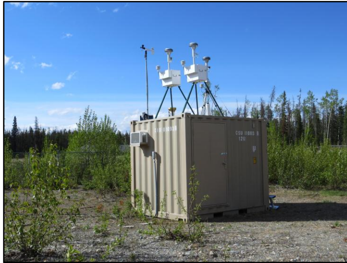
FIGURE 3.1. THE ENVIRONMENTAL ENCLOSURE AT TSAY KEH THAT HOUSES THE TEOM, DATALOGGING INSTRUMENTS AND PROVIDES A PLATFORM FOR THE METEOROLOGICAL SENSORS AND THE TEOM INLET.
