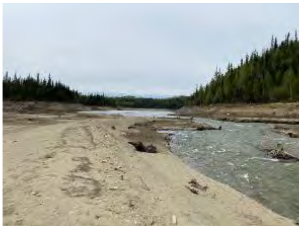
Figure 10 From left to right: Berm A; Berm F and Berm G (in background) with embedded LWD (Six Mile Creek, May 28, 2020).
