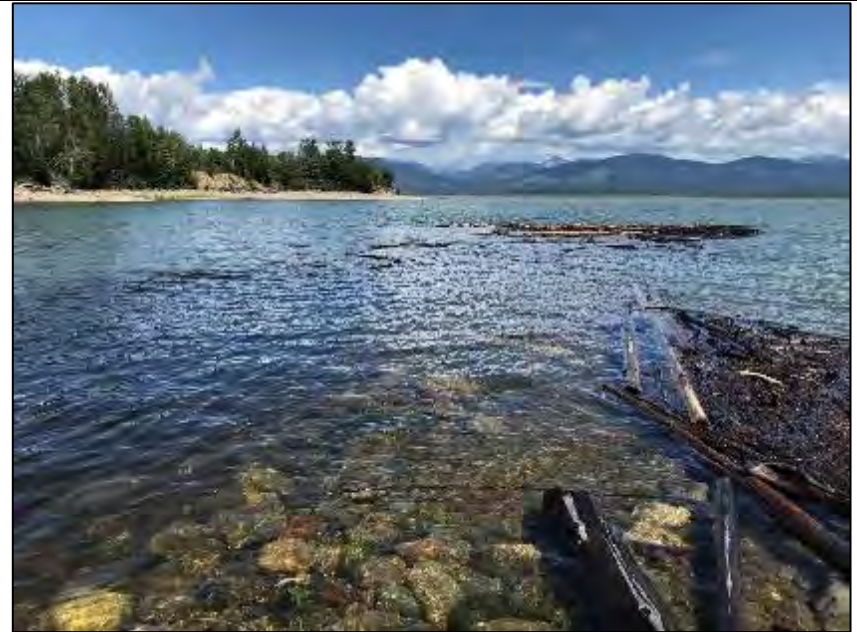
Photo D-1. Berm D – Berm D looking downstream. Date taken: July 4, 2020.
