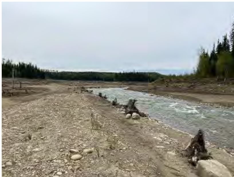
Figure 11 From left to right: Berm B with embedded LWD; Berm C with embedded stakes and rock spur; (Six Mile Creek, May 28, 2020).
