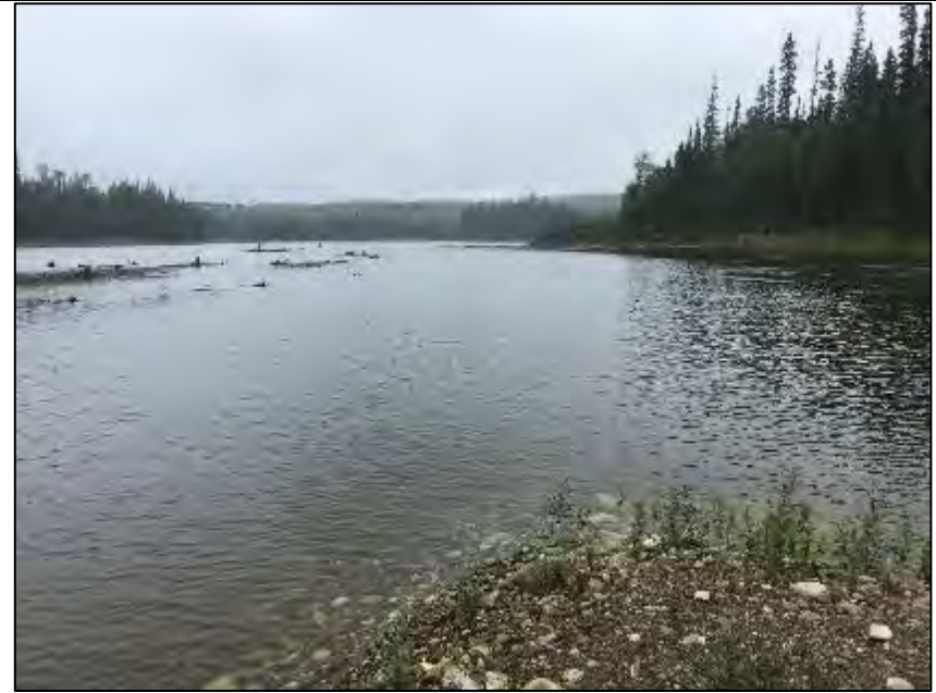
Berm D/F was fully submerged at the time of the site visit in 2020. Photo taken at the downstream end of Berm C.
