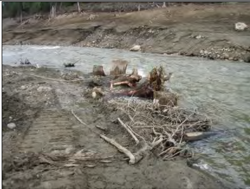
Photo A-1. Berm A with water level just below crest elevation. Date taken: May 22, 2014.
