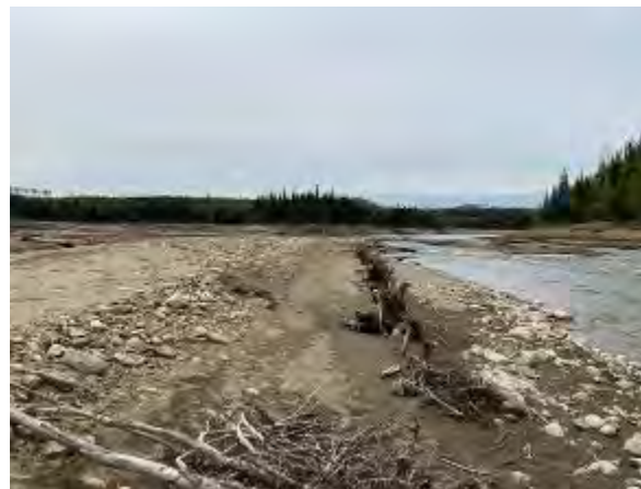
Figure 10 From left to right: Berm A; Berm F and Berm G (in background) with embedded LWD (Six Mile Creek, May 28, 2020).
