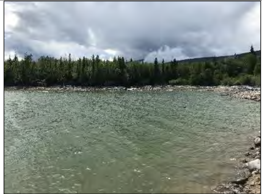
Photo B-1. Berm B – Site overview showing part of berm A, berm B, and most of berm C. Date taken: July 4, 2020.
