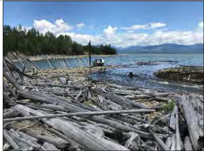
Photo A-1. Berm A – Downstream end of berm A, ECM use above EL. 671.0 m. Date taken: July 4, 2020.
