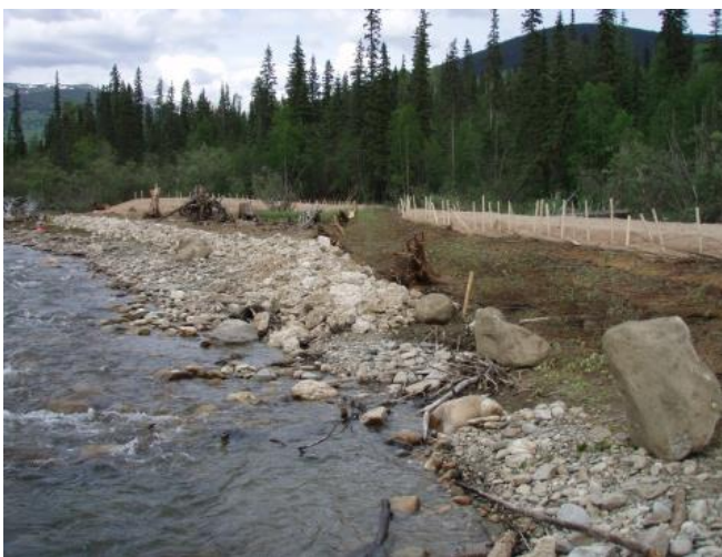
Braided channels and reshaping project at Six Mile Creek.
