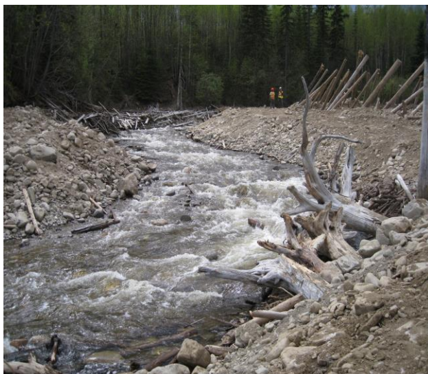
Debris plug and debris trap project at Ole Creek.
