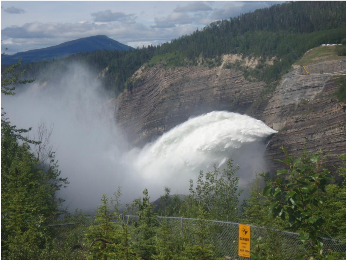
Figure 3. Spillway discharge (~1,477 cms) from the W.A.C. Bennett Dam, June 28 th . Photo credit: Kim Hawkins, BC Hydro.
