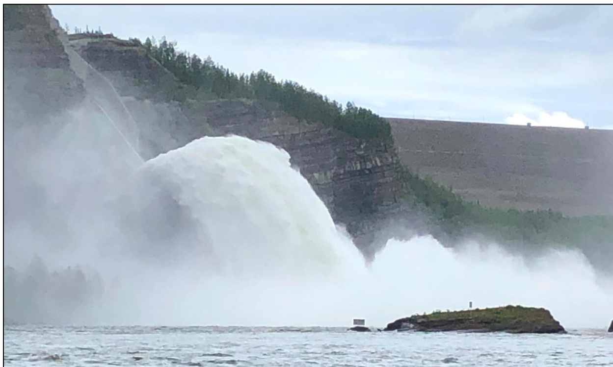
Figure 2. WAC Bennett Dam Spillway, July 17, 2020; 570 cms.
