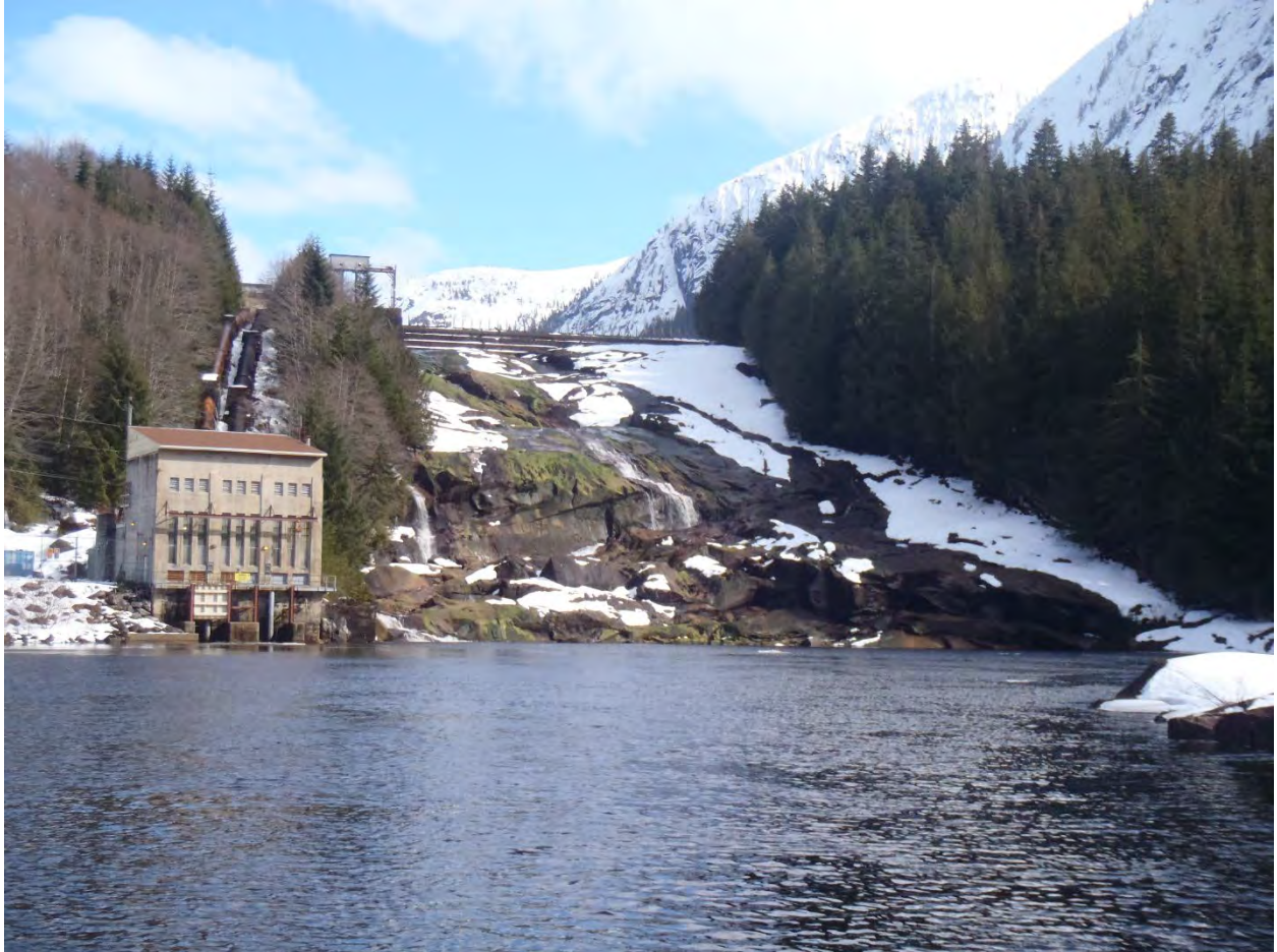
Falls River Generating Station and Dam (A. Hall 2011).
