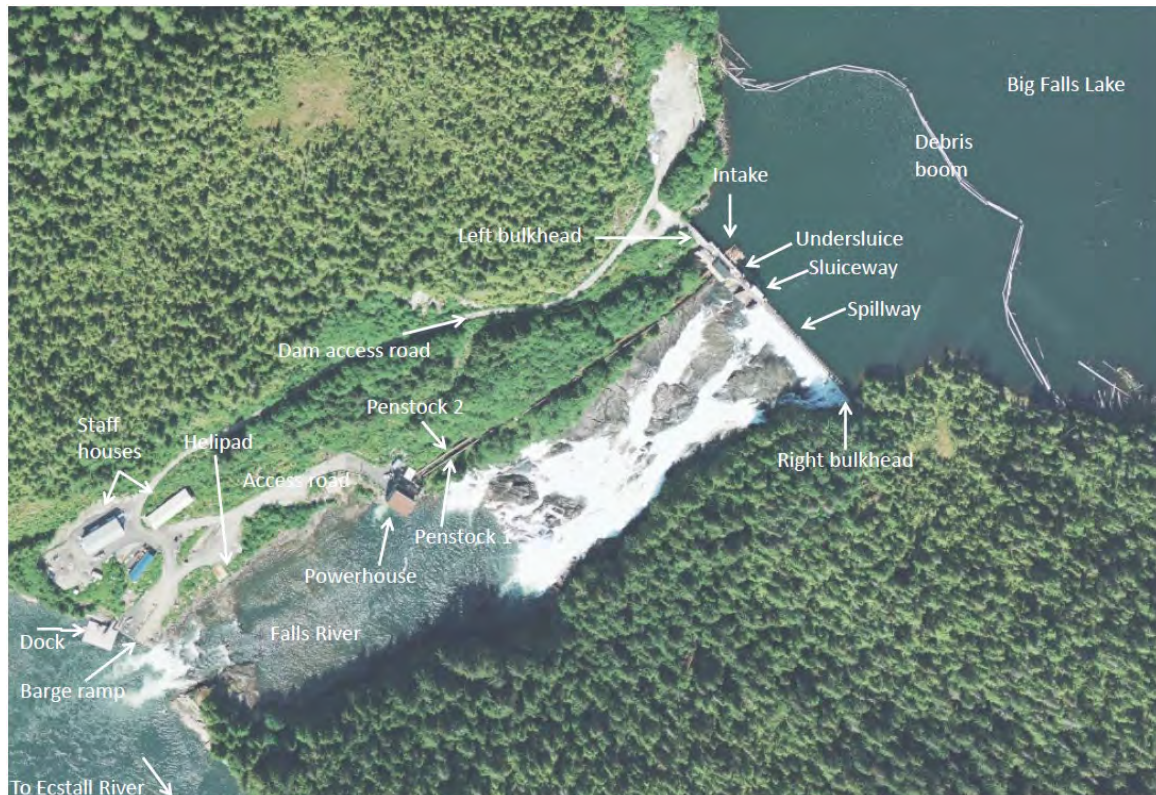
Figure 2.2. Falls River Dam and Downstream Components
