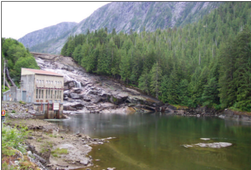
Photo 2-1: Falls River powerhouse and tailpond
