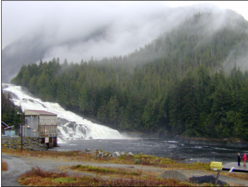
Photo 2-3: Falls River powerhouse with spill over falls during high inflows
