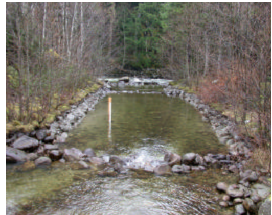
Photo 4-5: Tailrace Channel during Test Unit Shutdown, with 0.08 \text{ m}^3/\text{s} Minimum Flow provided through the Backup Water Supply Line (Photos taken by Ron Ptolemy, 29 January 2003)
