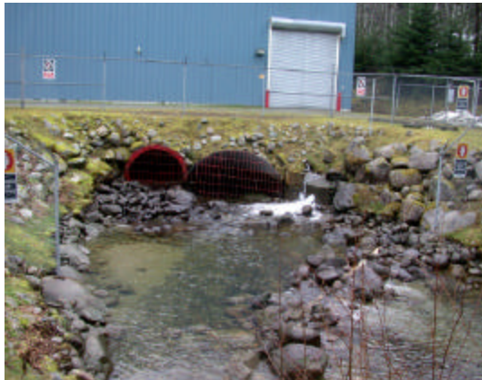
Photo 4-5: Tailrace Channel during Test Unit Shutdown, with 0.08 \text{ m}^3/\text{s} Minimum Flow provided through the Backup Water Supply Line (Photos taken by Ron Ptolemy, 29 January 2003)
