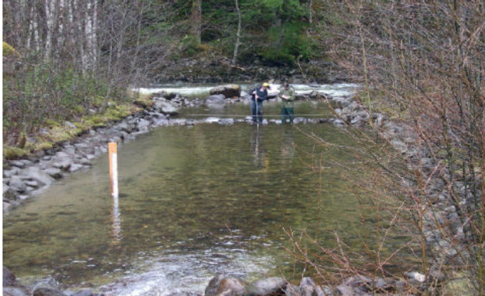
Photo 4-6: Powerhouse Tailrace Channel during Test Unit Shutdown, with 0.08 m 3 /s Minimum Flow provided through the Backup Water Supply Line. (Note sedimentation along right upstream bank)
