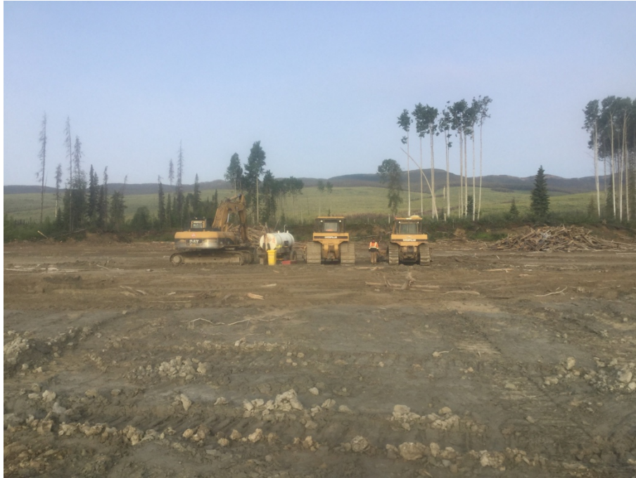
Figure 14: Refueling away from water with a spill kit next to refueling.
