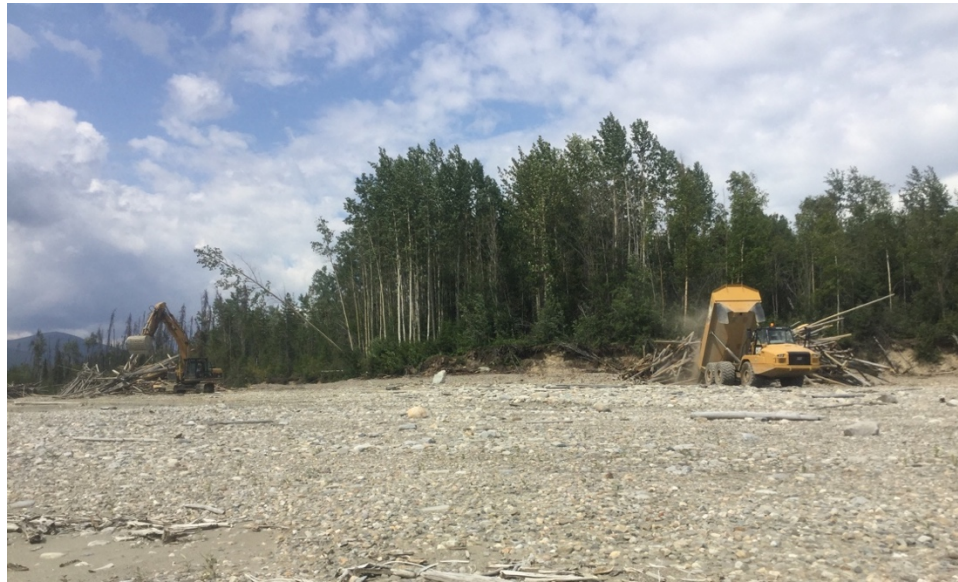
Figure 10: Debris piling by excavator and rock truck on Corless Beach.
