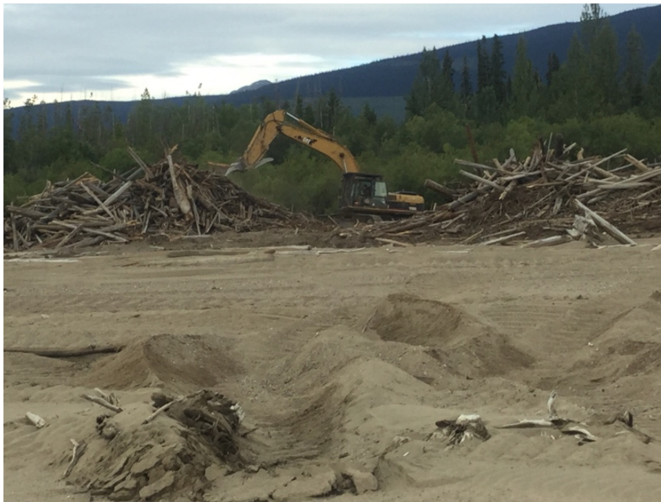
Figure 9: Excavator working on Corless A.
