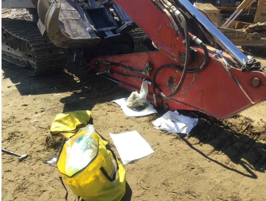
Figure 13: Repair of hydraulic line with attention to spill potential.
