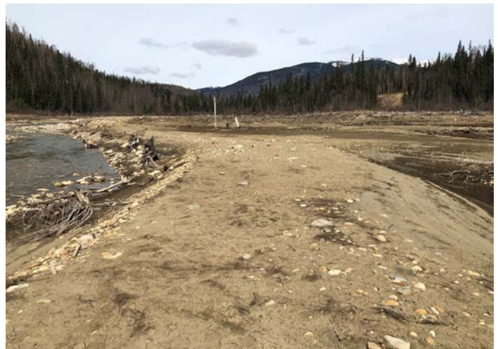
PHOTO 22: Upstream End of Berm 'F' Looking Upstream (repeat of 2016 Ph#15)
