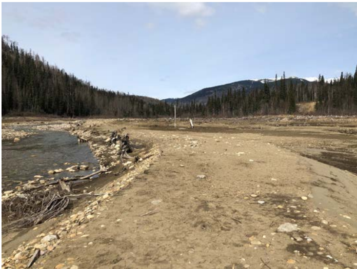
PHOTO 29: Looking Upstream at Berm 'D' (repeat of 2016 Ph#22)
