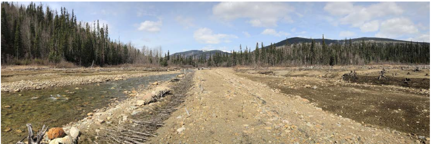
PHOTO 40 (Panoramic): Berm 'C' looking upstream from downstream end (repeat of 2016 Ph#31)
