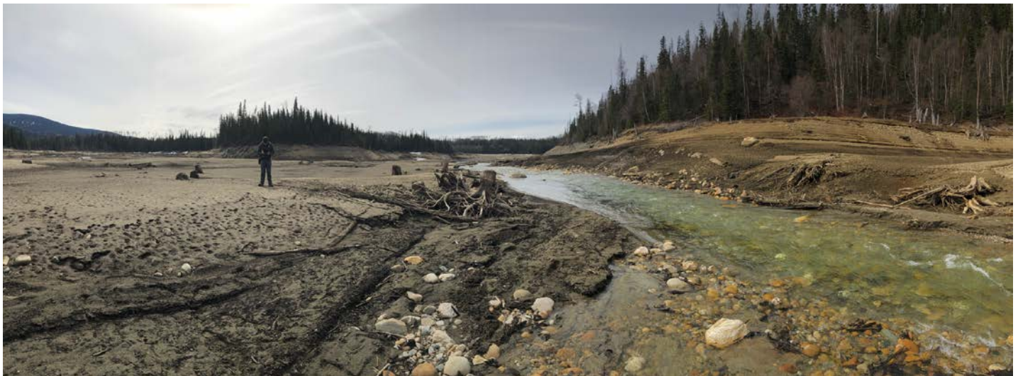
PHOTO 6 (Panoramic): Looking Downstream at Berm 'A'
