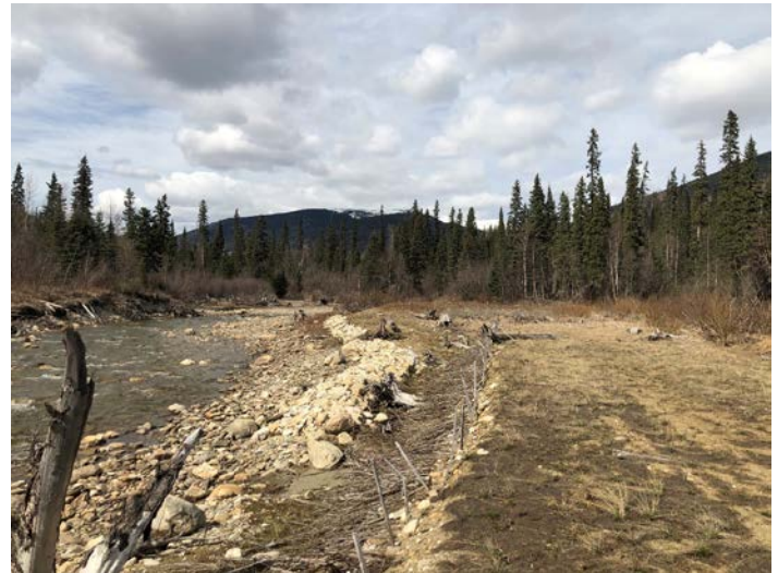
PHOTO 50: Looking upstream at upstream end of Berm 'C' (repeat of 2016 Ph#41)
