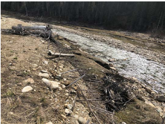
PHOTO 45: Coir soil wraps, willow brush layers along berm and native grasses/reeds at toe (repeat of 2016 Ph#36)
