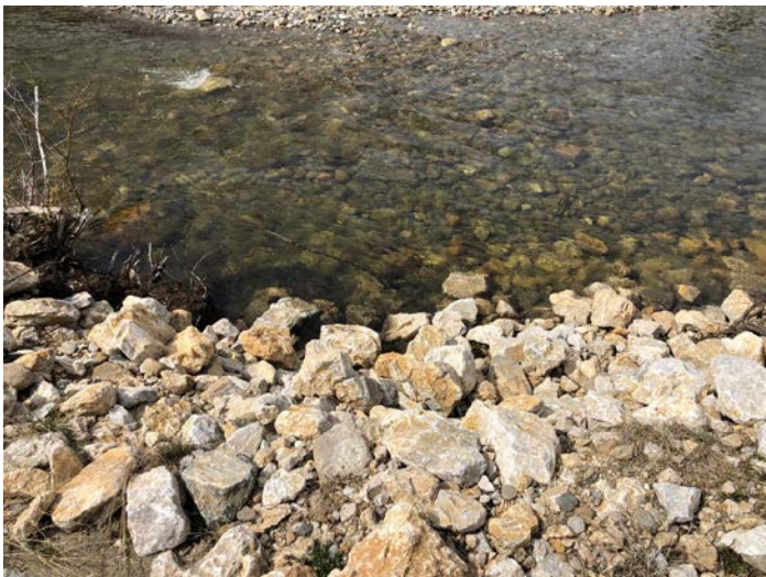
PHOTO 59: Launching riprap toe (repeat of 2016 Ph#48)
