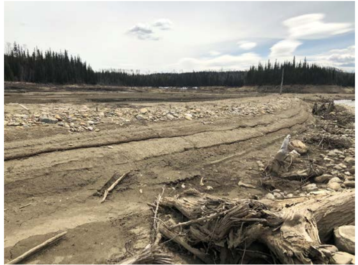
PHOTO 26: Coir Geogrid "Soil Wrap" Layers in Good Condition. Note Upper Layer is ECM (repeat of 2016 Ph#19)
