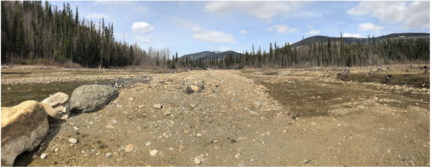
PHOTO 39 (Panoramic): Downstream end of Berm 'C' looking upstream (repeat of 2016 Ph#30)
