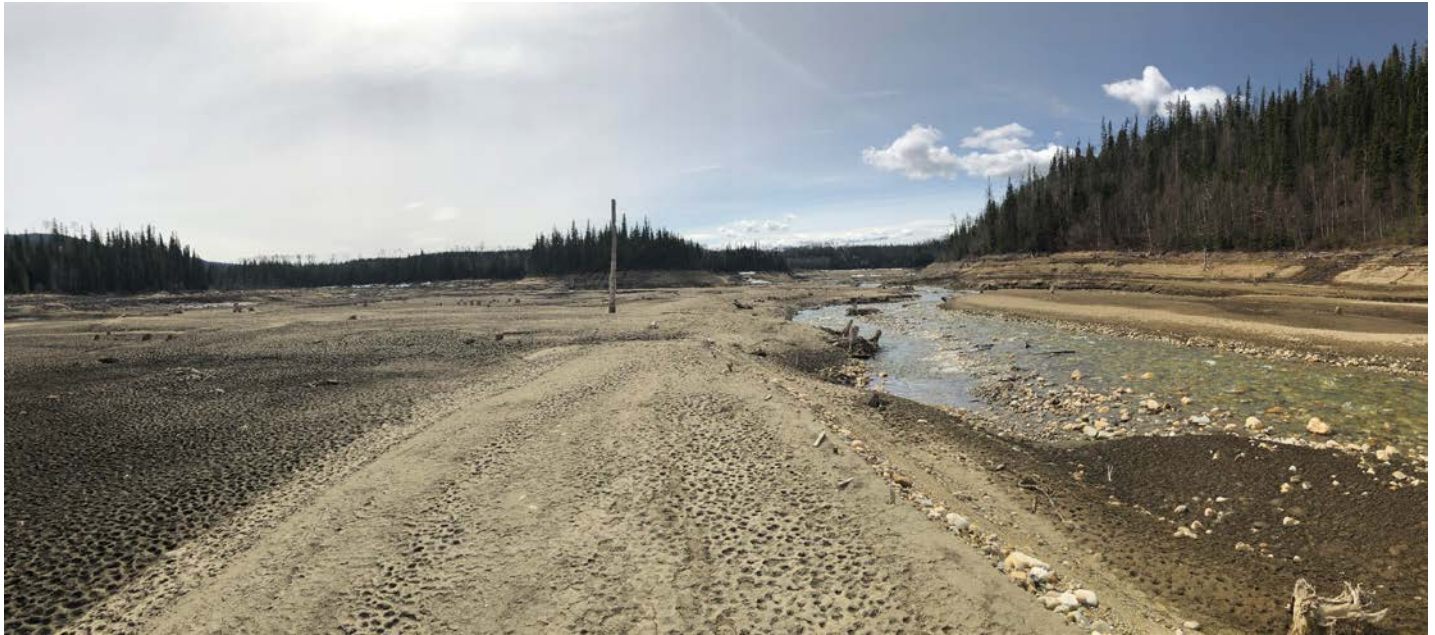
PHOTO 10: Looking Downstream at Berm 'A' and Berm 'G' (repeat of 2016 Ph#6)
