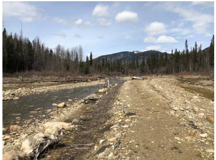
PHOTO 44: Downstream end of Berm 'C' looking upstream (repeat of 2016 Ph#35)
