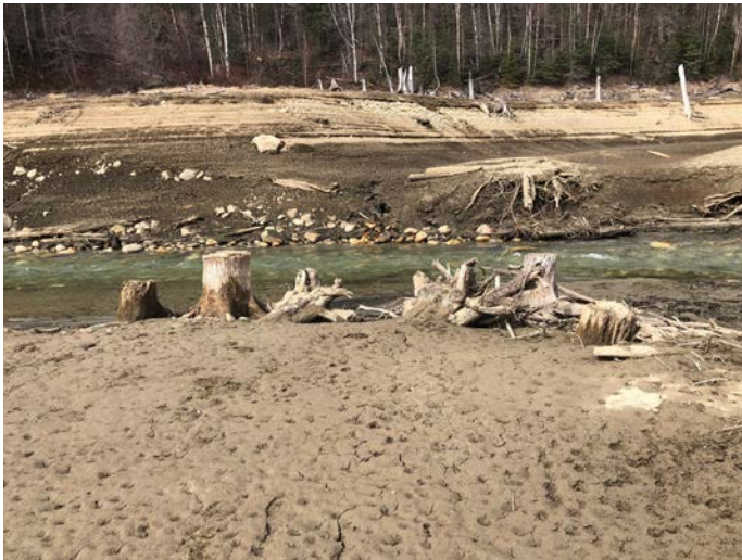
PHOTO 8: Looking at Berm 'A' from Left Bank
