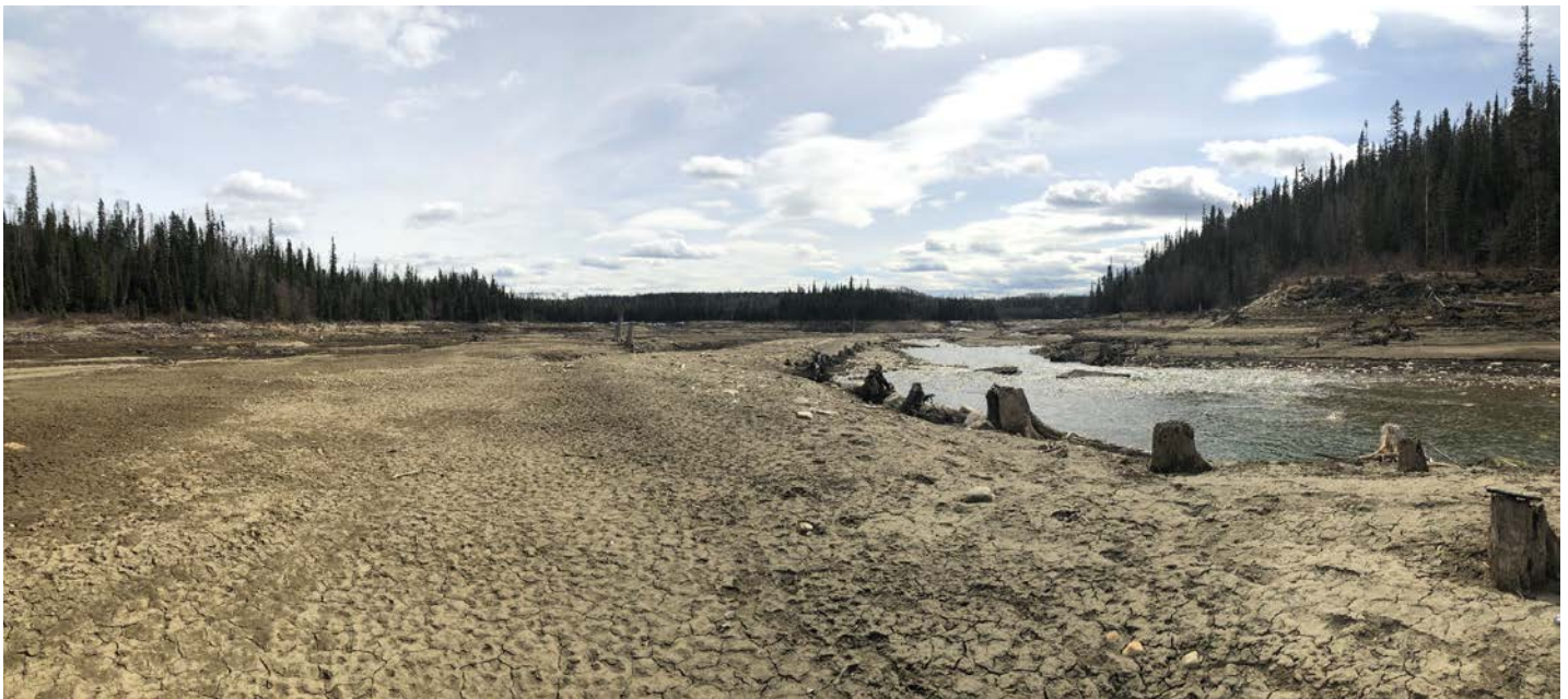
PHOTO 27 (Panoramic): Looking Downstream at Berm 'D' (repeat of 2016 Ph#20)
