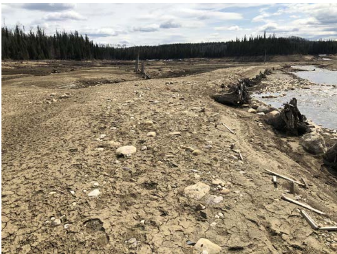
PHOTO 31: Material Used to Cover ECM When it Became Buoyant Still in Place, also Deposition (repeat of 2016 Ph#24)
