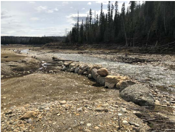
PHOTO 43: Downstream end of Berm 'C' looking downstream (repeat of 2016 Ph#34)
