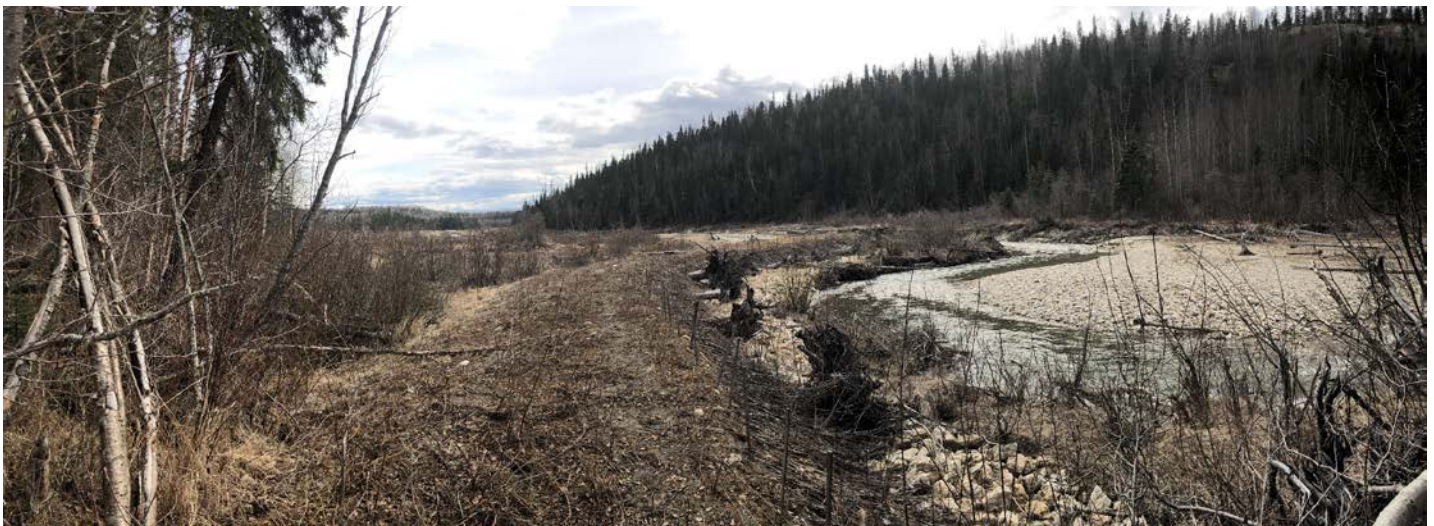
PHOTO 53 (Panoramic): Looking downstream at Berm 'J' (repeat of 2016 Ph#44)
