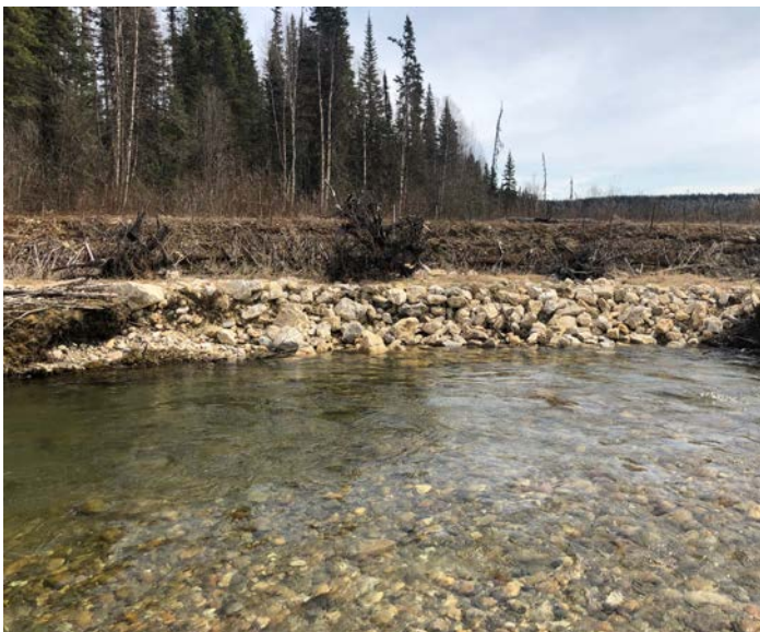
PHOTO 65: Launched Toe Riprap at Berm 'J'
