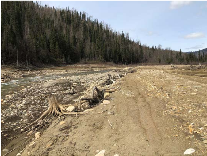
PHOTO 35: Coir Soil Wraps in Good Condition (repeat of 2016 Ph#28)
