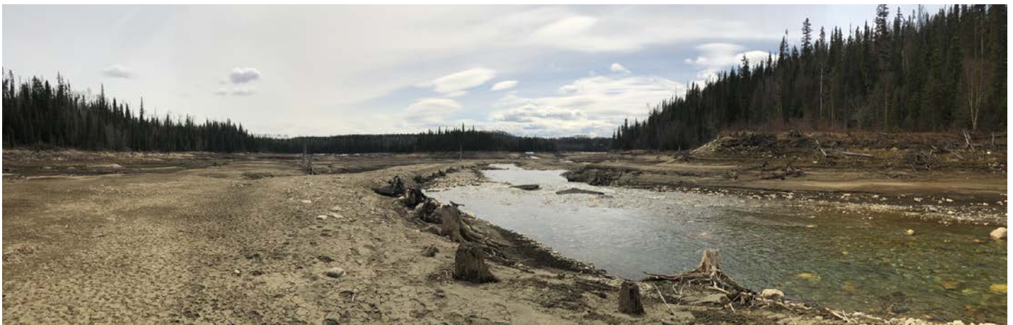
PHOTO 16 (Panoramic): Looking Downstream at Berms 'D' and 'F'
