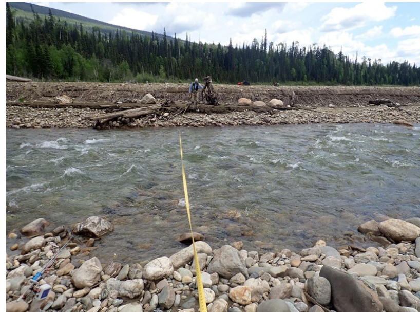
Figure 11 From left to right: Berm J with embedded LWD, sprouting embedded stakes and sprouting willow stakes on berm crest; discharge measurement site (Six Mile Creek, June 13, 2018)
