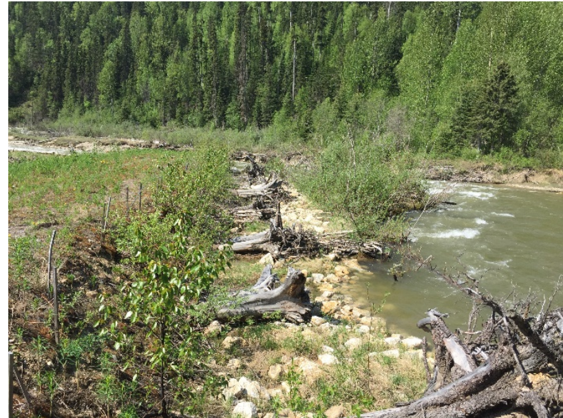
Figure 11 From left to right: Berm J with embedded LWD on June 13, 2018 (left picture) and on May 28, 2019 (right picture).
