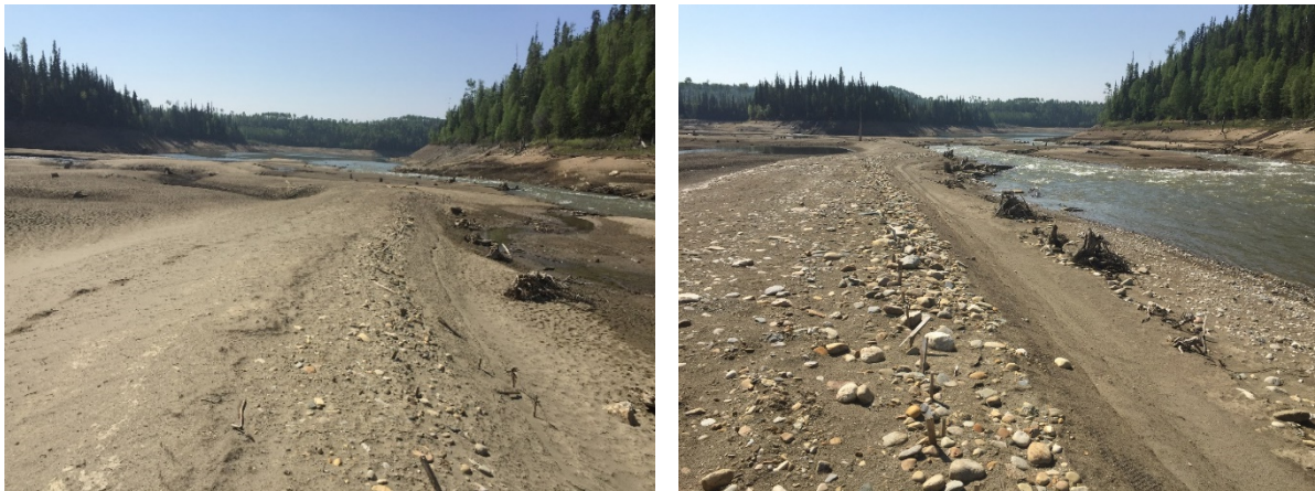
Figure 9 From left to right: Berm A; Berm F and Berm G (in background) with embedded LWD (Six Mile Creek, May 28, 2019).
