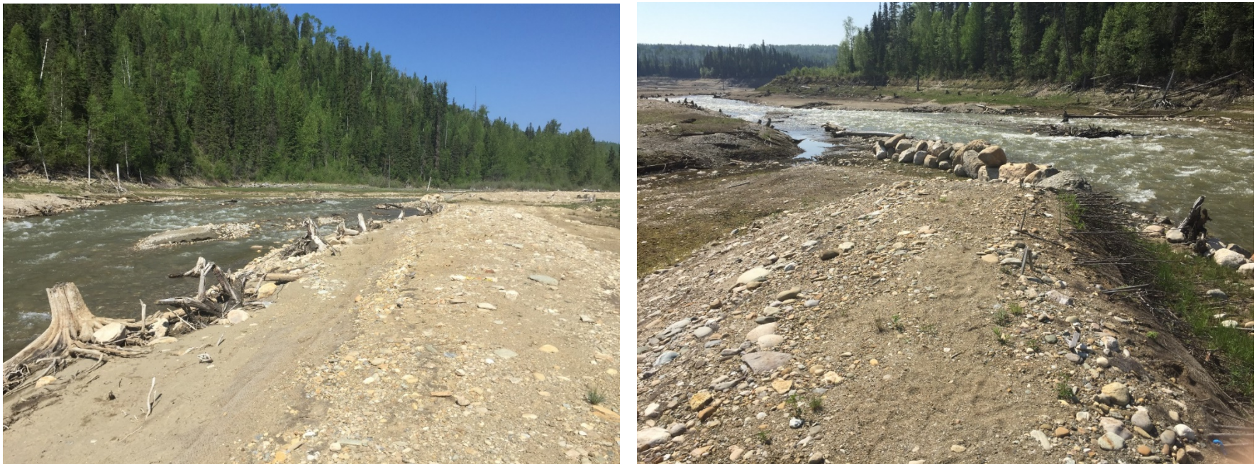
Figure 10 From left to right: Berm B with embedded LWD; Berm C with embedded stakes and rock spur; (Six Mile Creek, May 28, 2019).
