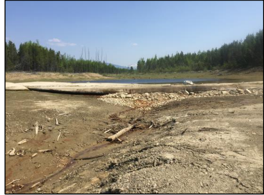
Image 14: Looking upstream from the Beaver Pond impoundment (May 26, 2019).
