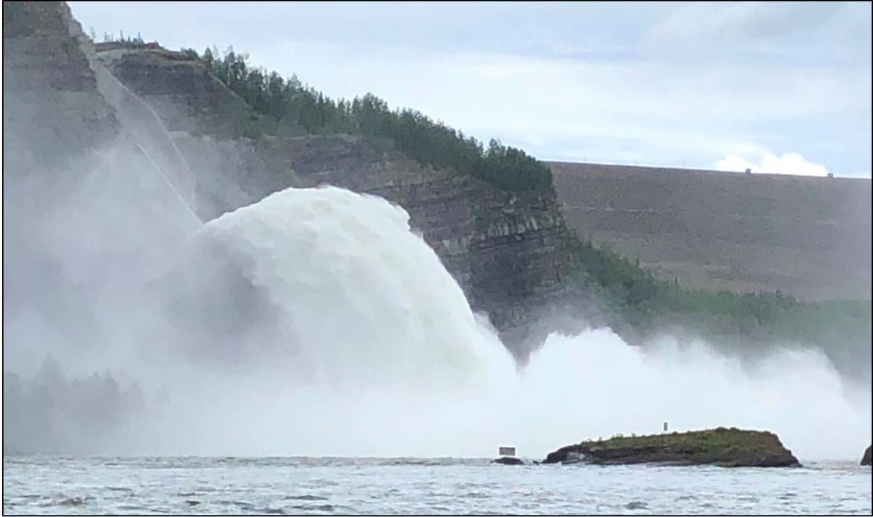
Figure 2. WAC Bennett Dam Spillway, July 17, 2020; 570 cms.
