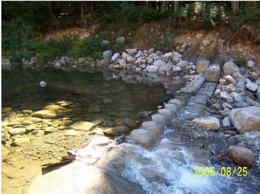
**Figure 5.1.b. Replacement Boulder Creek Newbury style weir, October 2015 (BC Hydro 2016).**
