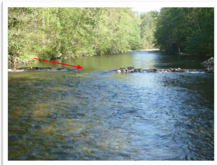
Figure 10 - Index site 2a - upstream view of weir, Sept.09.13 Discharge = 2.65cms (WSC Port Coquitlam) The arrow identifies breached access point over weir.
