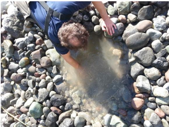
**Photo 1: Excavating sediment for sediment trap installation.**
