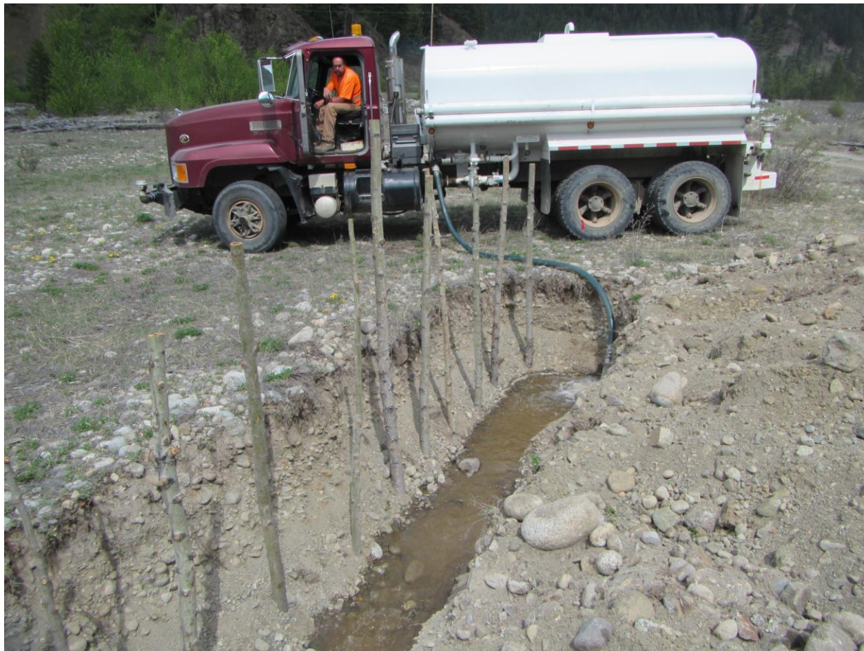
Figure 4 Watering cuttings trenches on the Gun Creek Fan West, prior to backfilling with excavator. 20 April 2016
