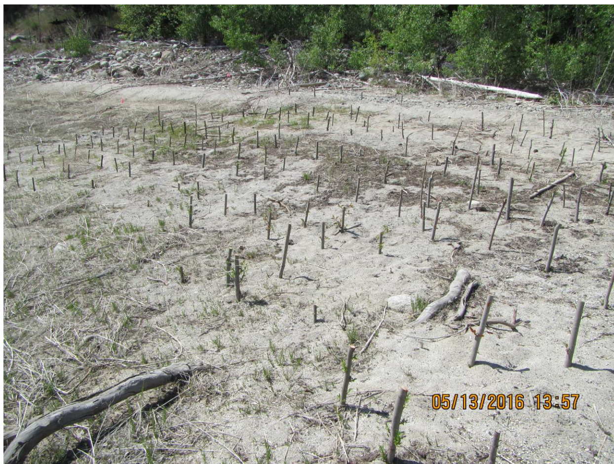
Figure 11 SHB west end polygon of live stake cuttings photographed 13May 2016 a month after planting , green shoots are noted sprouting from the stakes.
