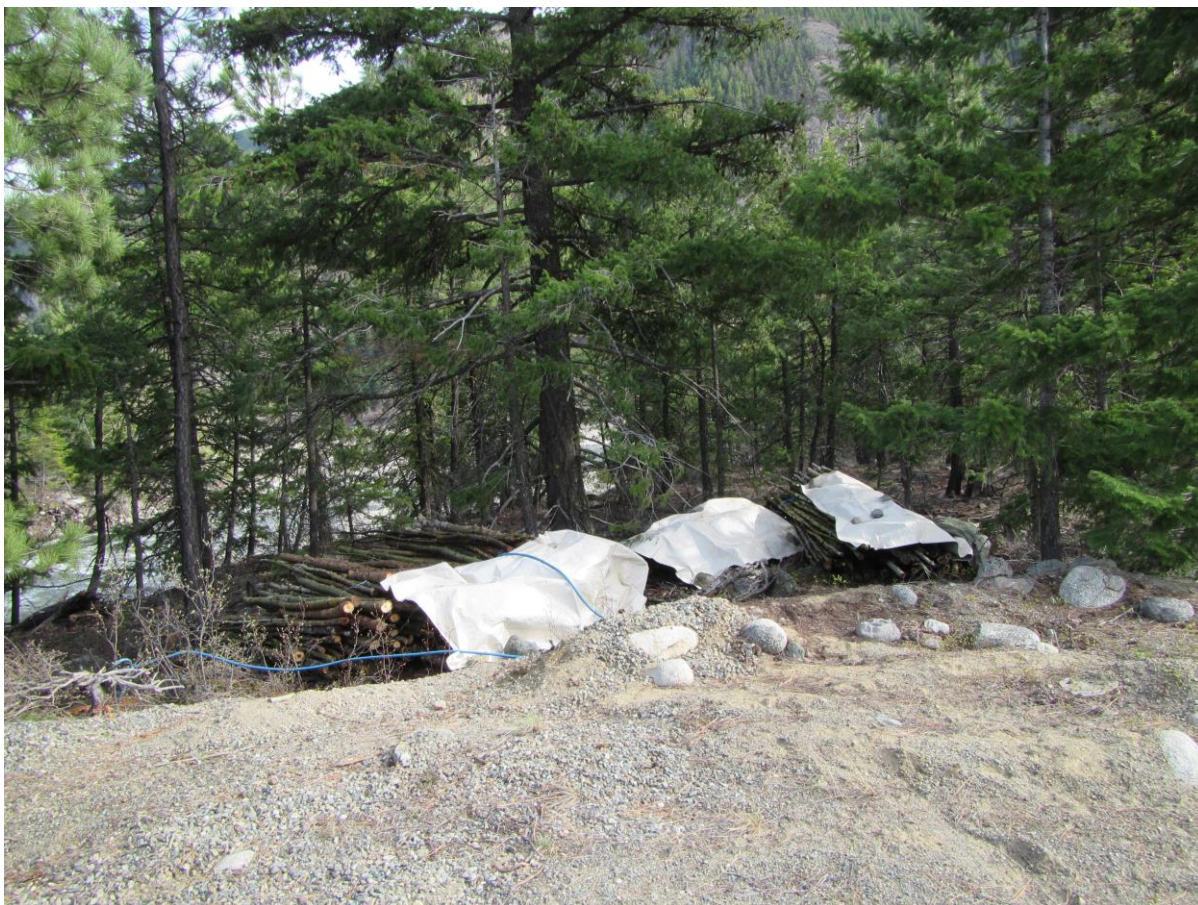
Figure 1 live stake cutting staged on the GCFW just prior to planting. 13 May 2016
