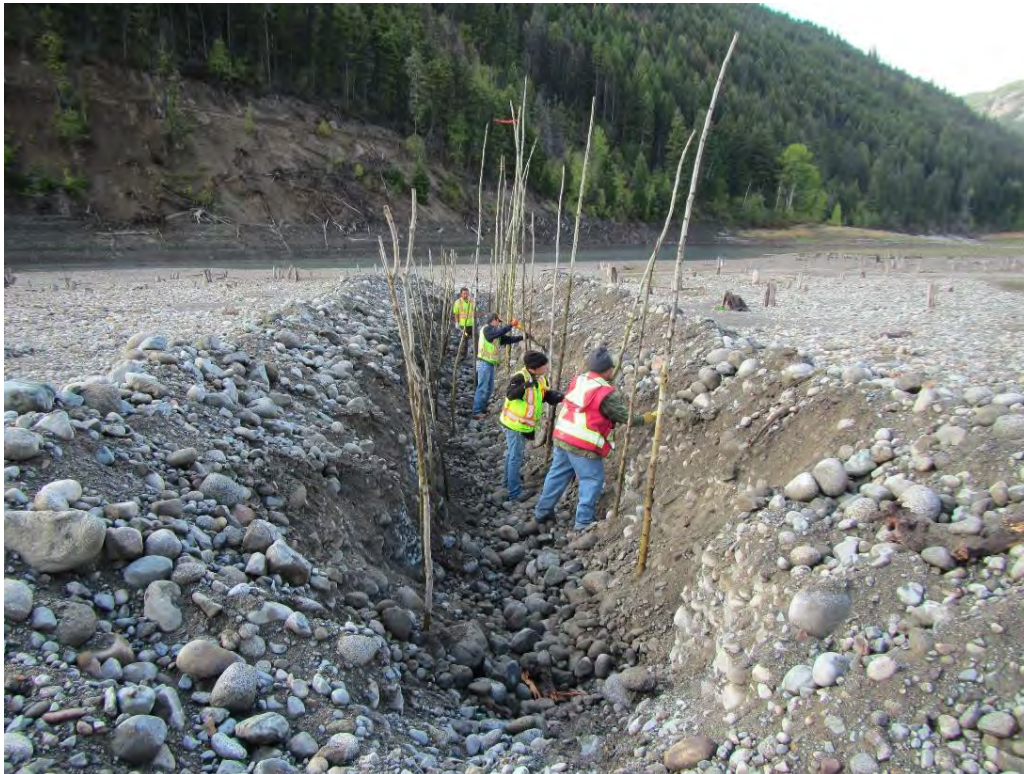
Figure 6 Planting cottonwood cuttings in machine-dug trench on the Gun Creek Fan 05 May 2015.
